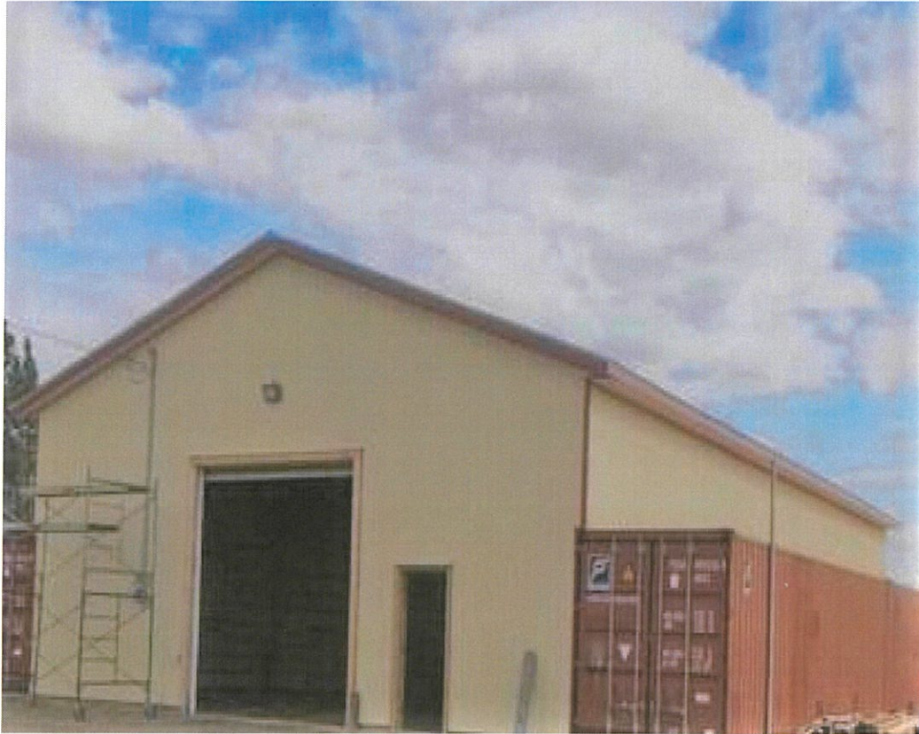
Core Box Storage Building
