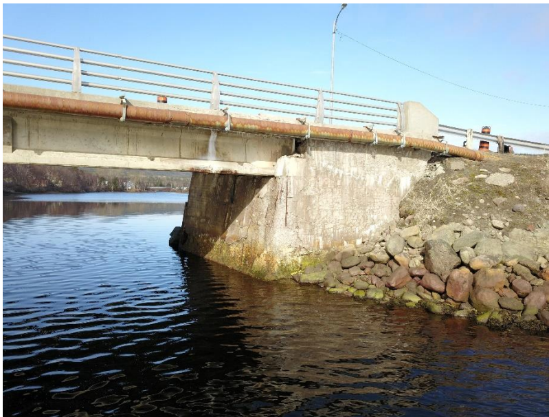
Photo 4 – Northern abutment of current bridge facing west
