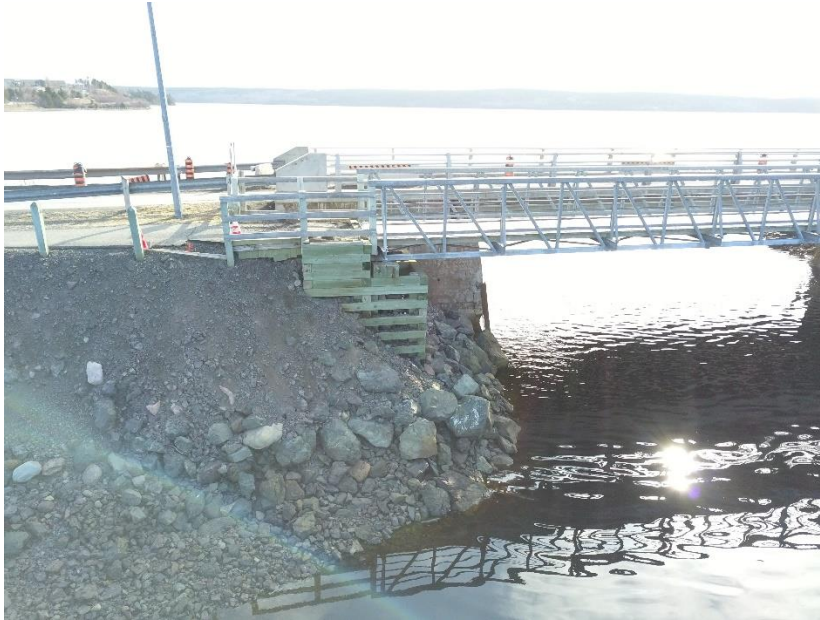
Photo 3 – Northern abutment of current bridge facing east.
