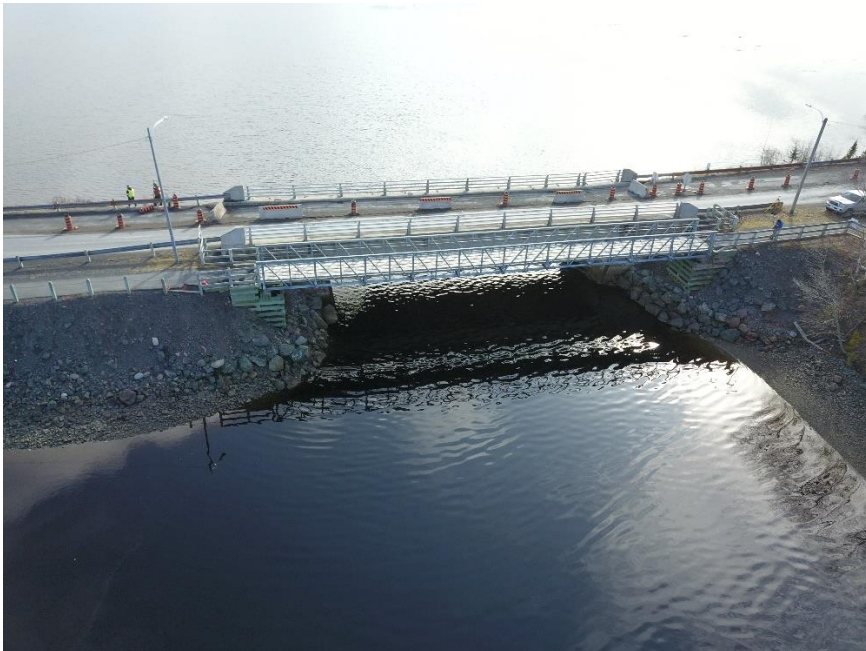
Photo 2 – Current bridge structure facing east.
