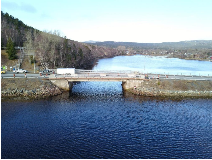
Photo 1 – Drone imagery of current bridge structure facing west.
