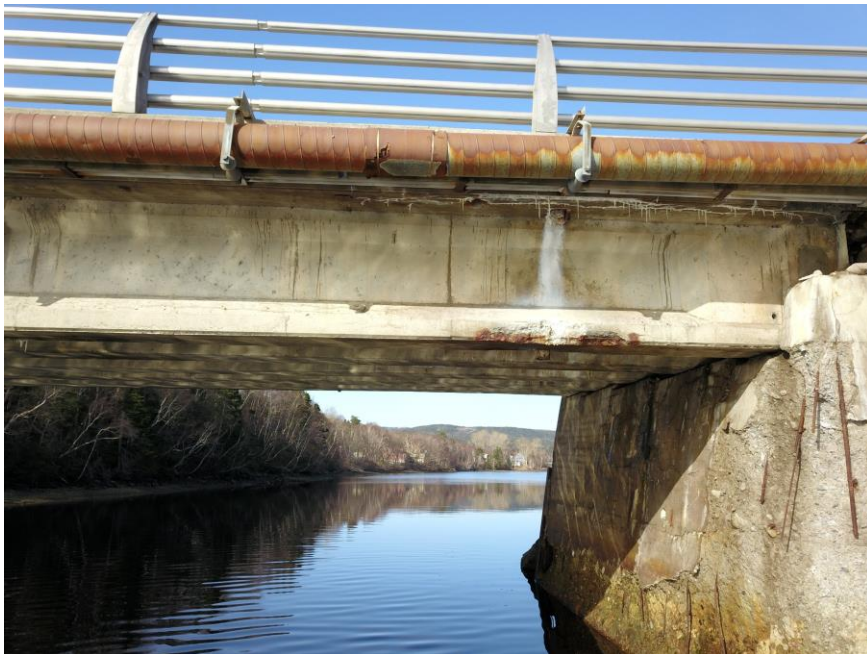
Photo 6 – Close view of the east side of the bridge.
