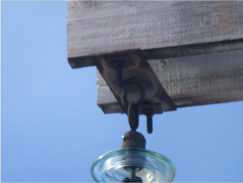
Figure A-7: Worn Ball Link Eye Bolt
