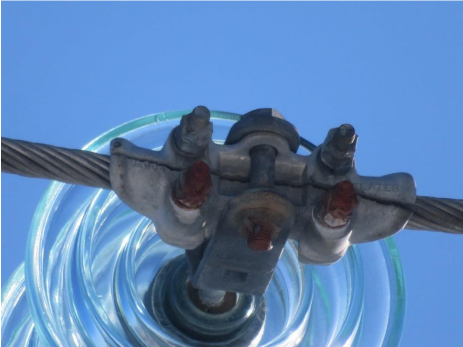
Figure A-6: Split FlexAll Clamp
