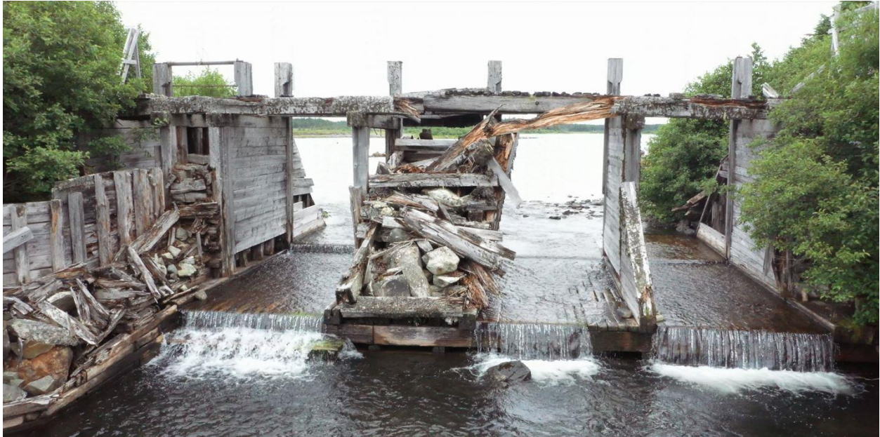
Figure 2.3 Long Lake WCS – Facing Upstream
