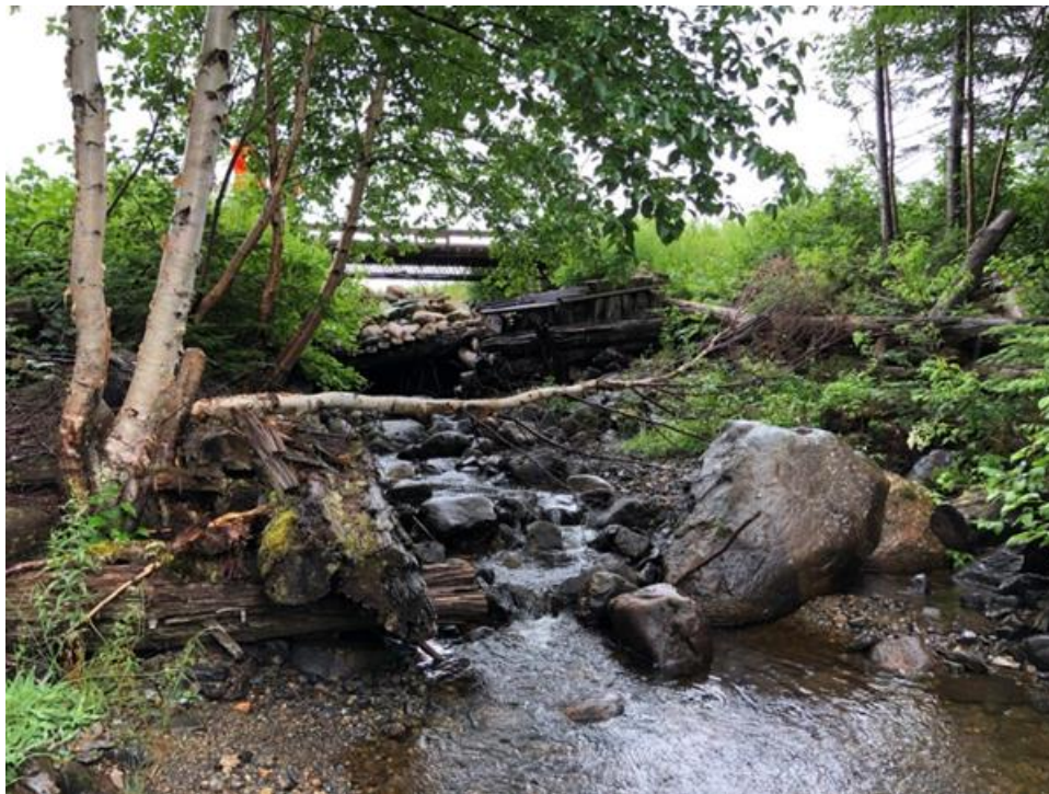
Figure 2.7 Shoulder Blade Lake WCS Facing Upstream
