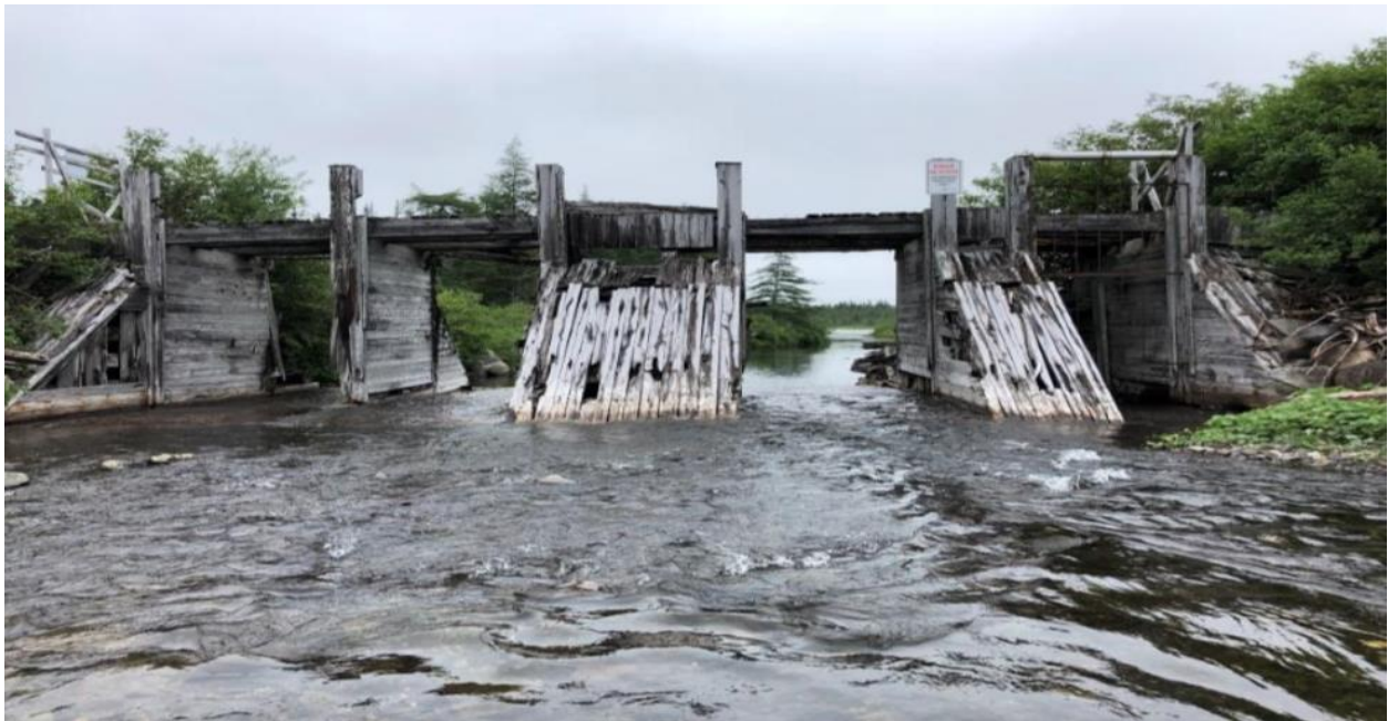
Figure 2.4 Long Lake WCS – Facing Downstream
