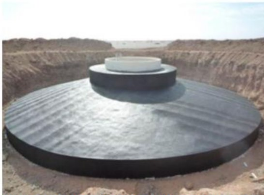
Figure 2.35 Example of a Shallow Matt Foundation with Concrete Poured Prior to Backfilling
