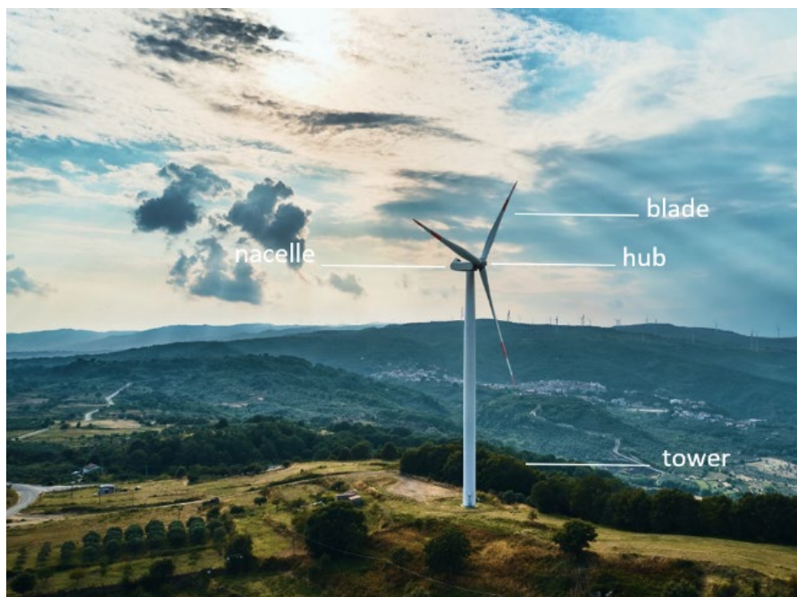
Figure 2.8 Typical Wind Turbine Components
