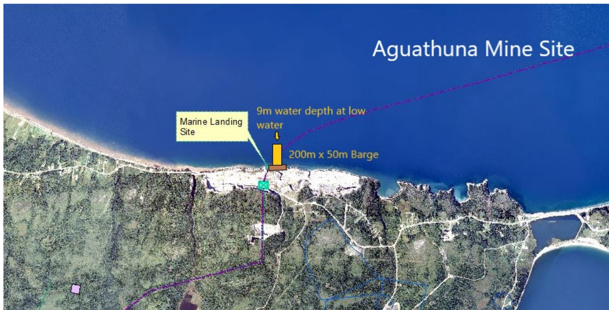
Figure 3.3 Possible Barge Landing: Aguathuna Site
