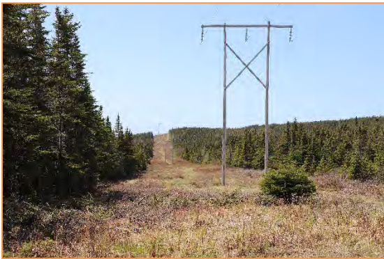
Examples of an H Frame Transmission Line and Substation on the Port au Port Peninsula.
