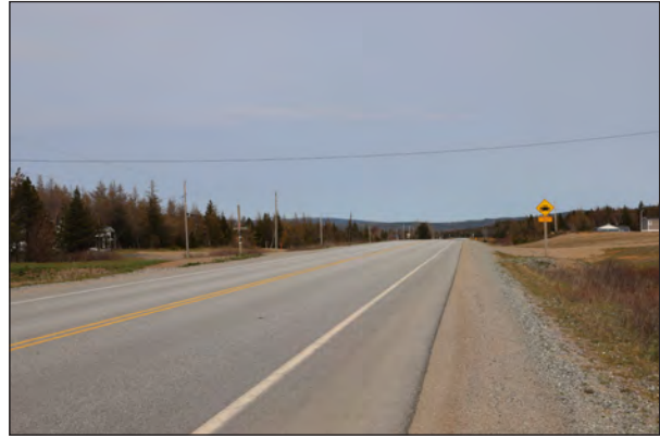
VP C19 - Trans Canada Highway Potential Visible Project - Codroy Wind Farm Northwest View (Stantec Image 200-0124)
