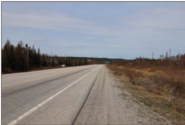
VP T15 - Trans Canada Highway Potential Visible Project - T-Line Southwest View (Stantec Image 85-9829)
