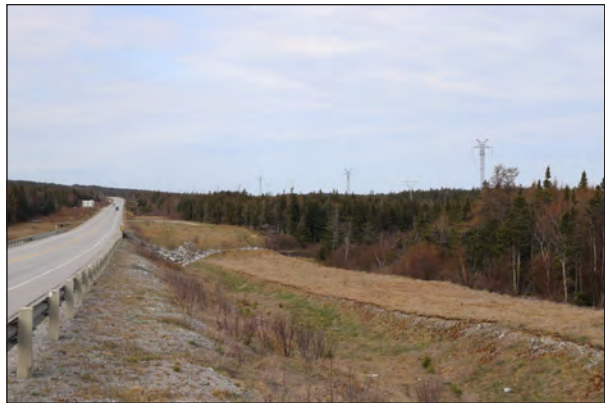
VP T10 - Trans Canada Highway Potential Visible Project - T-Line Southwest View (Stantec Image 78-9736)
