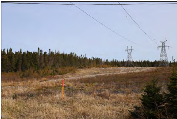
VP T17 - Trans Canada Highway Potential Visible Project - T-Line North View (Stantec Image 88-9861)
