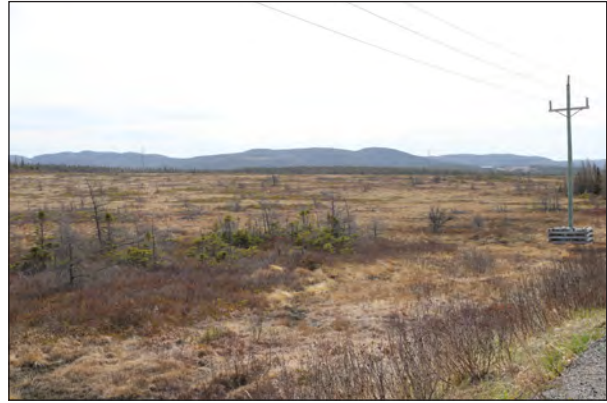
VP T14 - Steel Mountain Road Potential Visible Project - T-Line Northeast View (Stantec Image 83-9809)
