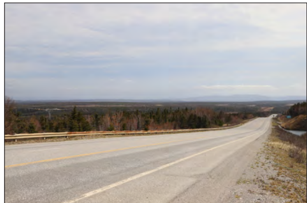
VP T18 - Trans Canada Highway Potential Visible Project - T-Line Southwest View (Stantec Image 91-9892)
