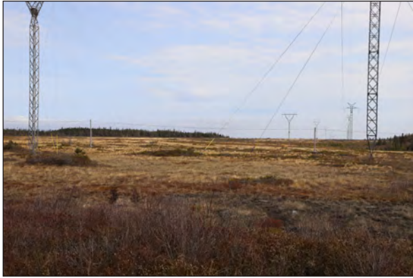
VP T13 - Steel Mountain Road Potential Visible Project - T-Line North View (Stantec Image 82-9783)
