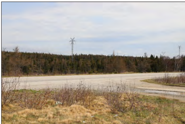
VP T11 - Trans Canada Highway Potential Visible Project - T-Line Northwest View (Stantec Image 81-9765)
