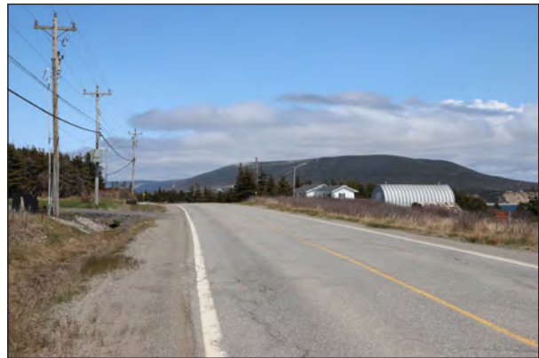
VP 50 - Route 460 Potential Visible Project - Port au Port Wind Farm / T-Line Northeast View (Stantec Image 49-9373)
