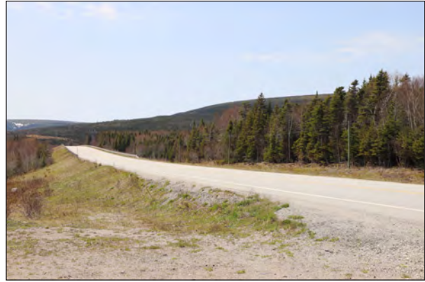
VP C13 - Trans Canada Highway Potential Visible Project - Codroy Wind Farm / T-Line West View (Stantec Image 193-0075)
