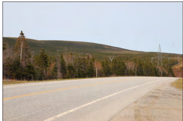
VP C23 - Trans Canada Highway Potential Visible Project - Codroy Wind Farm / T-Line Northeast View (Stantec Image 204-0172)
