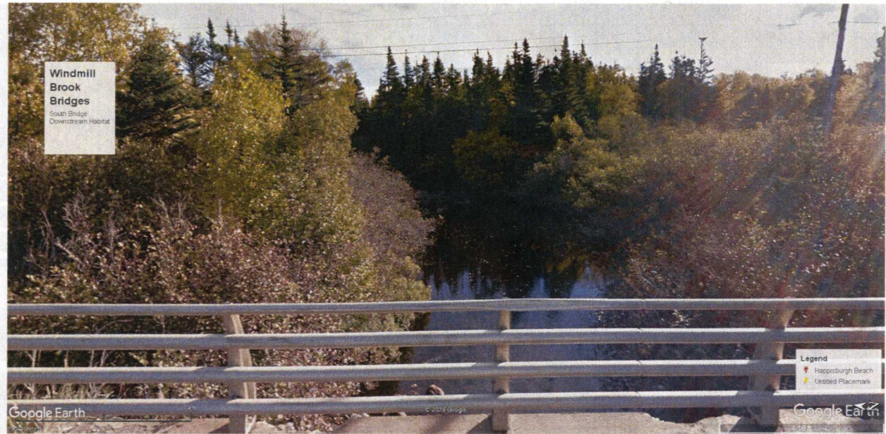
Fig. 6: Windmill Brook South Bridge Upstream
