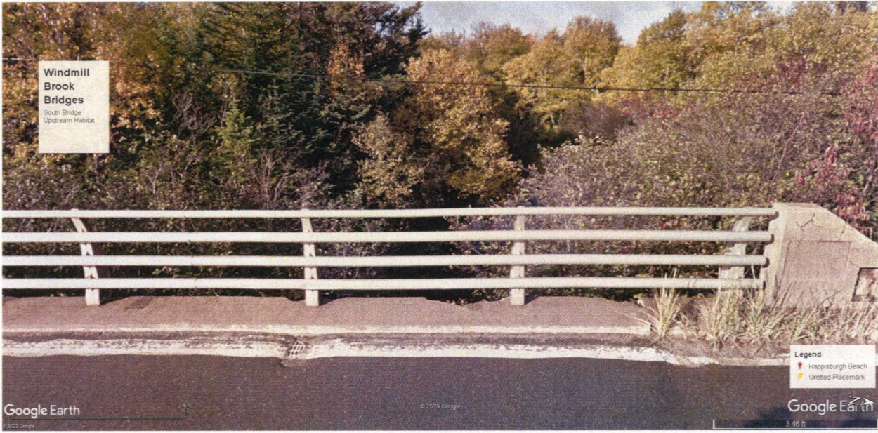
Fig. 6: Windmill Brook South Bridge Upstream
