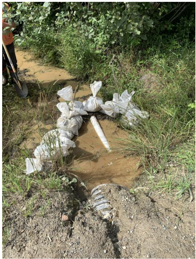
Figure 2 - Inverted Weir
