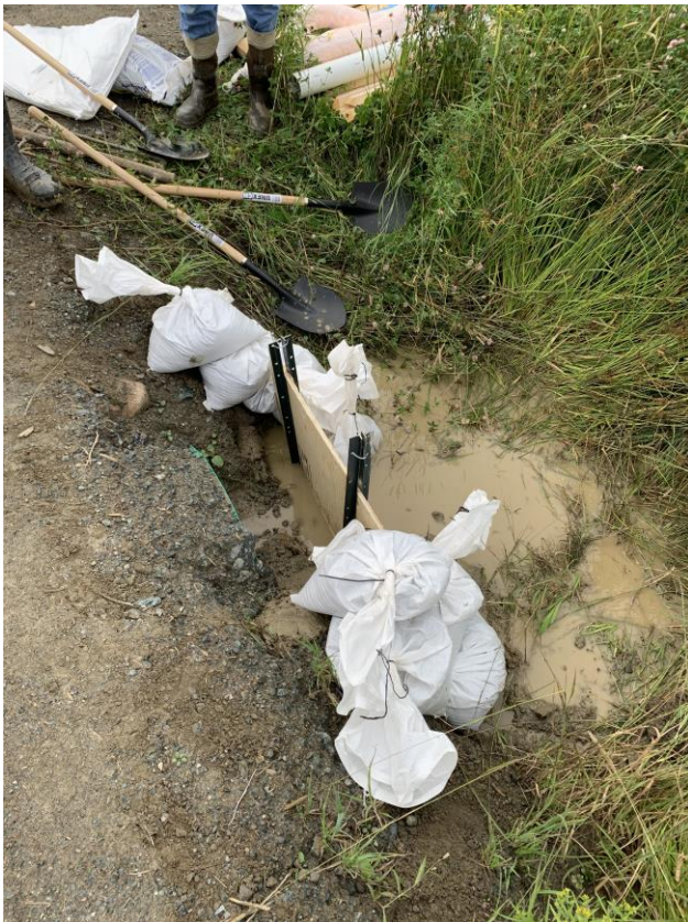
Figure 1 - Culvert Blocking
