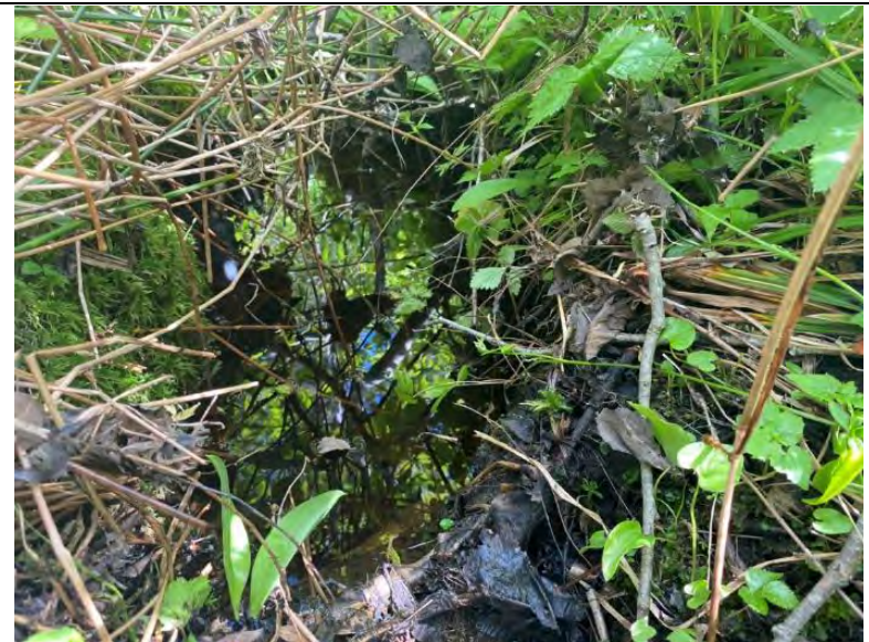
Photo 20 Watercourse Crossing WCF-1009 Facing Downstream
