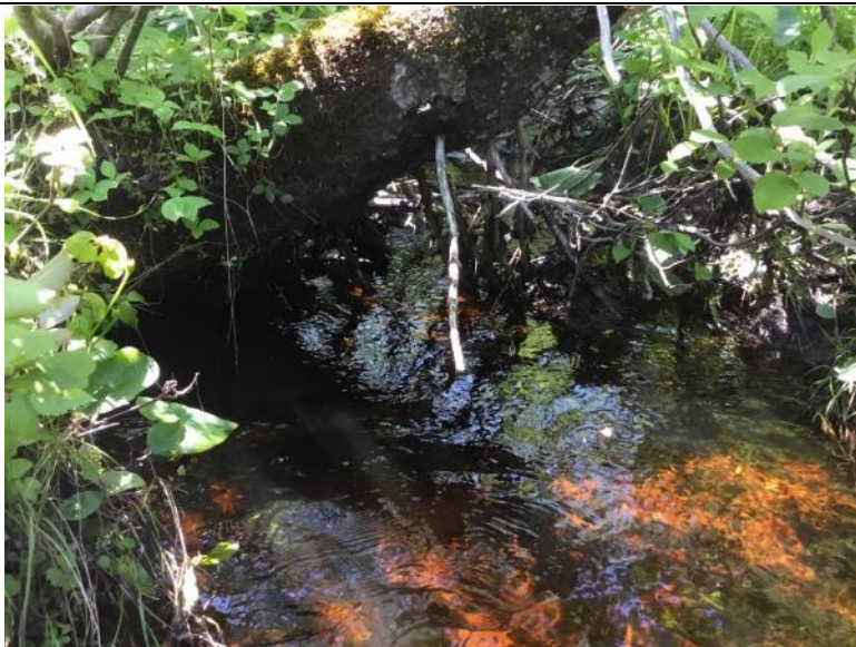
Photo 135 Watercourse Crossing WCA-111b Facing Upstream
