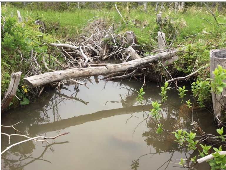
Photo 57 Watercourse Crossing WCA-057c Facing Upstream
