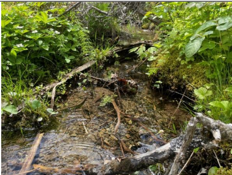
Photo 101 Watercourse Crossing WCA-073a Facing Upstream
