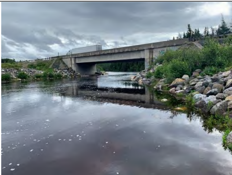
Photo 381 Watercourse Crossing WCT-574 Facing Upstream
