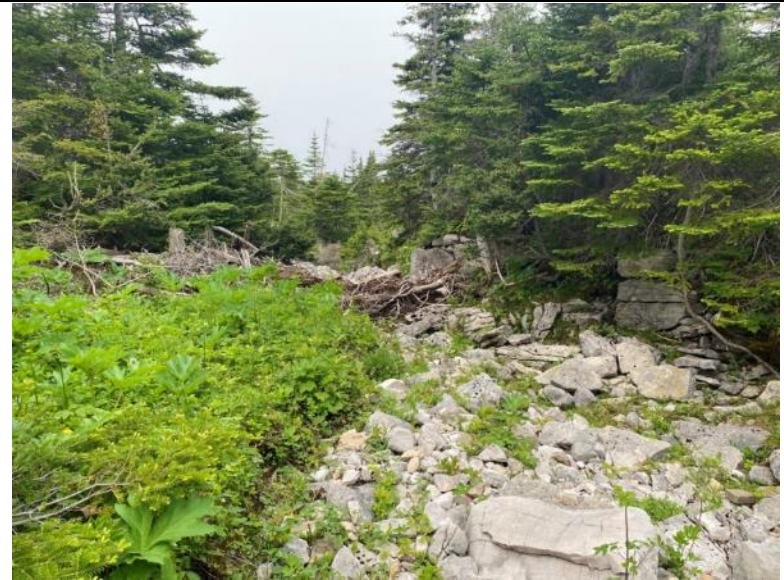
Photo 10 Watercourse Crossing WCA-011b Facing Downstream
