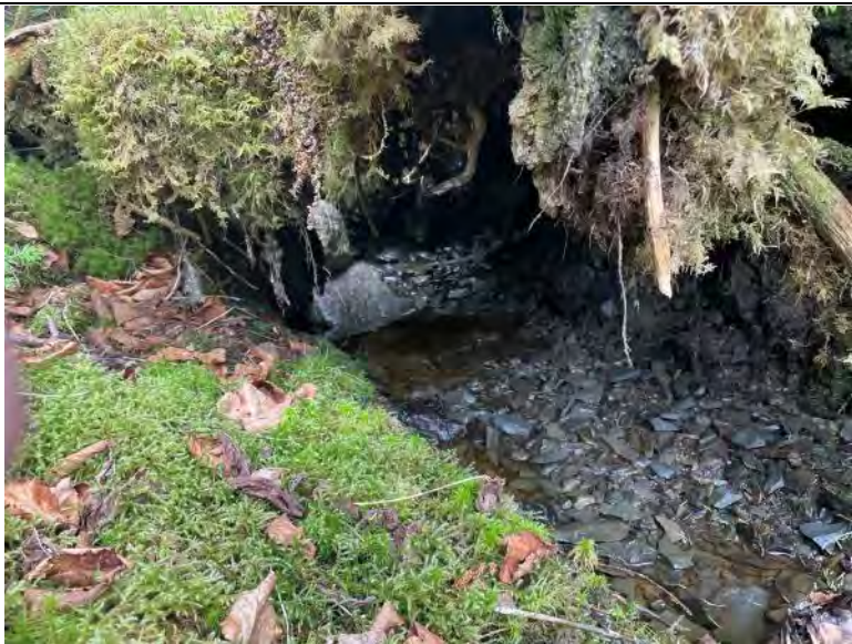
Photo 151 Watercourse Crossing WCL-769 Facing Upstream
