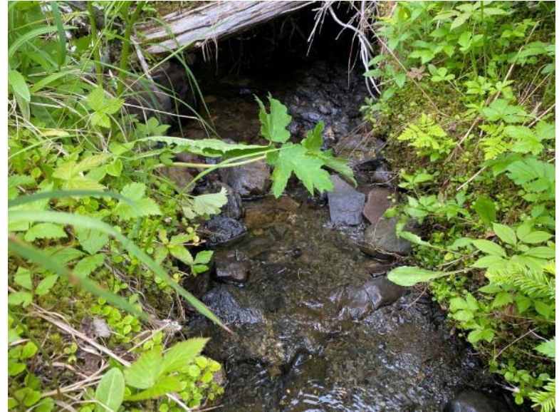
Photo 106 Watercourse Crossing WCA-074a Facing Downstream
