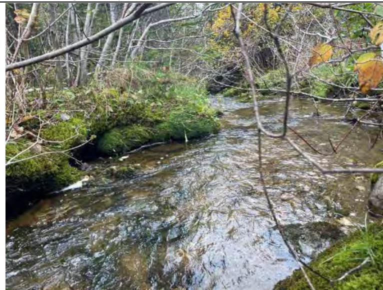
Photo 402 Watercourse Crossing WCT-630 Facing Downstream
