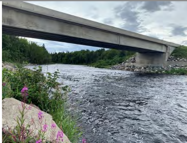
Photo 384 Watercourse Crossing WCT-583 Facing Downstream
