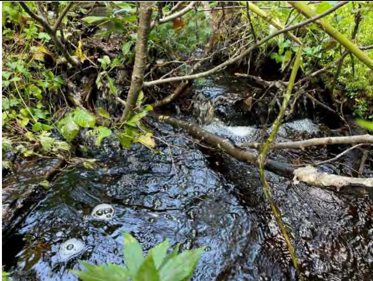
Photo 213 Watercourse Crossing WCL-895 Facing Upstream
