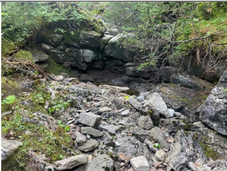
Photo 171 Watercourse Crossing WCA-132 Facing Upstream
