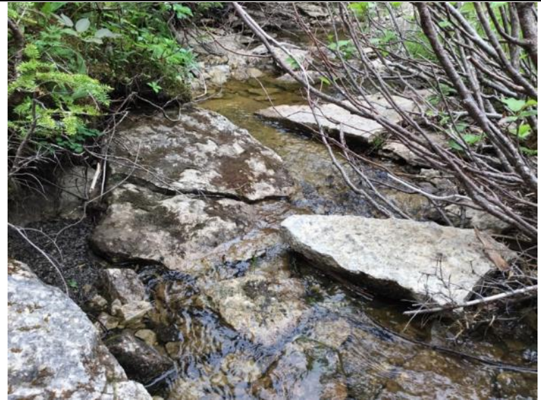
Photo 62 Watercourse Crossing WCA-057e Facing Downstream
