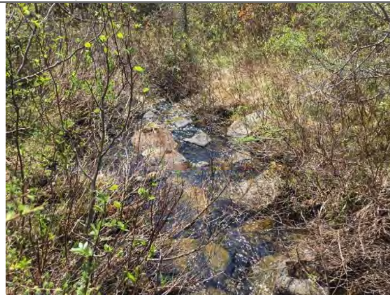
Photo 318 Watercourse Crossing WCT-518 Facing Downstream
