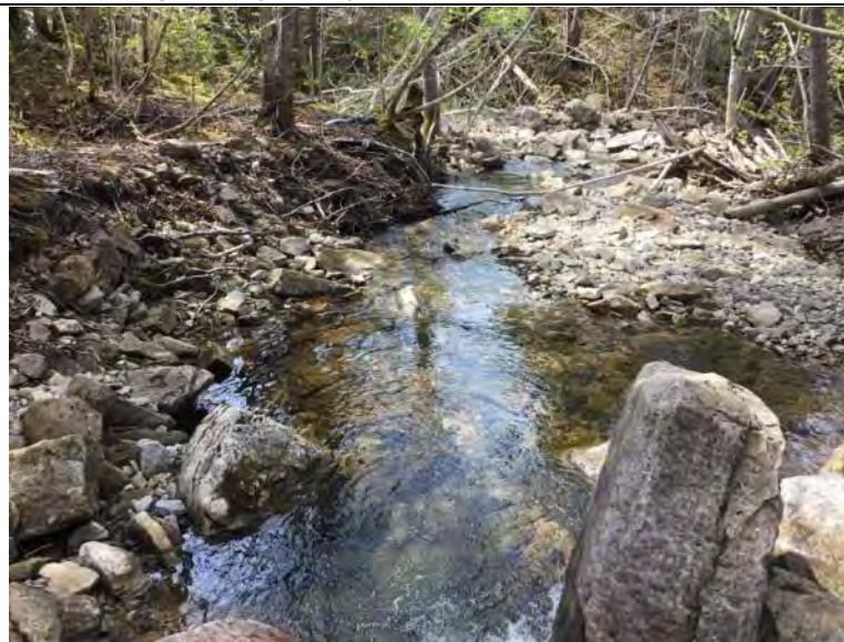
Photo 314 Watercourse Crossing WCT-515 Facing Downstream
