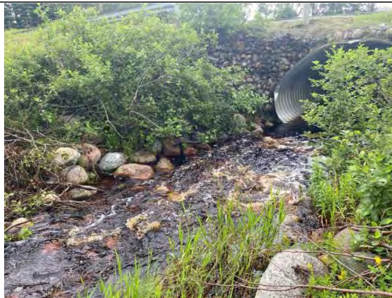
Photo 376 Watercourse Crossing WCT-549 Facing Downstream
