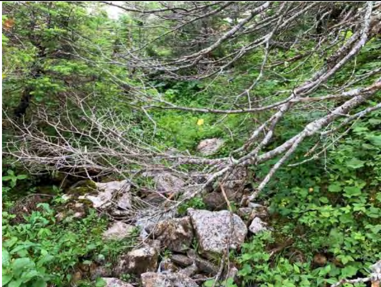
Photo 219 Watercourse Crossing WCL-896d Facing Upstream
