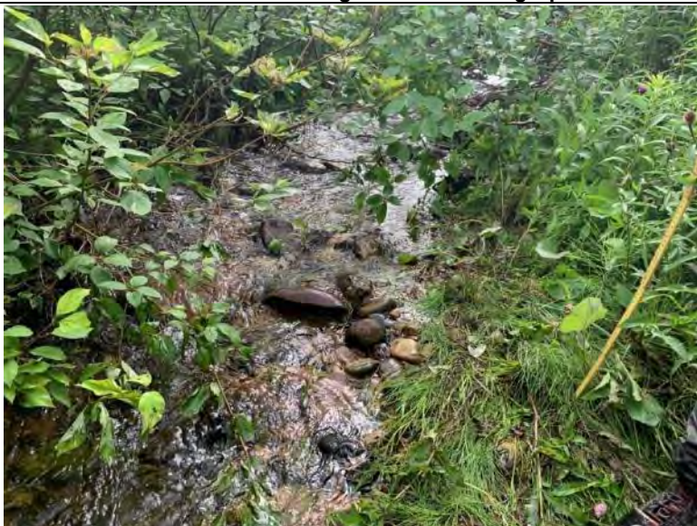
Photo 407 Watercourse Crossing WCT-633 Facing Upstream
