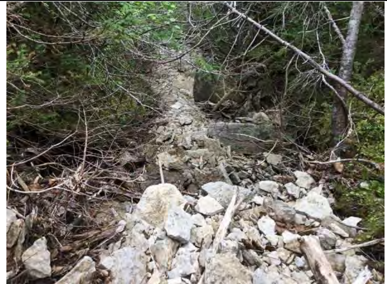
Photo 204 Watercourse Crossing WCL-867 Facing Downstream
