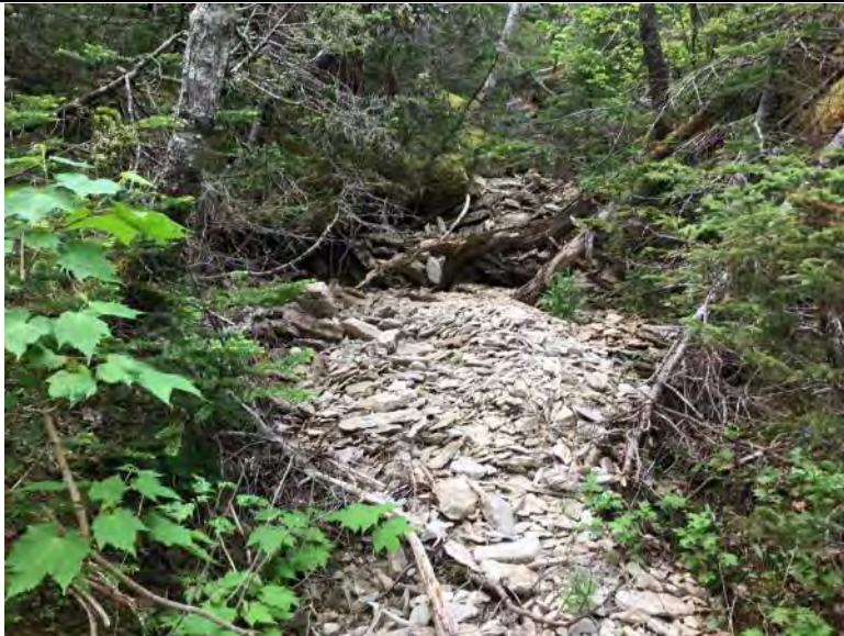
Photo 203 Watercourse Crossing WCL-867 Facing Upstream
