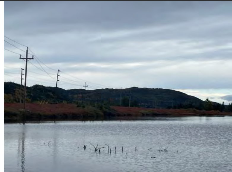
Photo 362 Watercourse Crossing WCT-537 Facing Downstream
