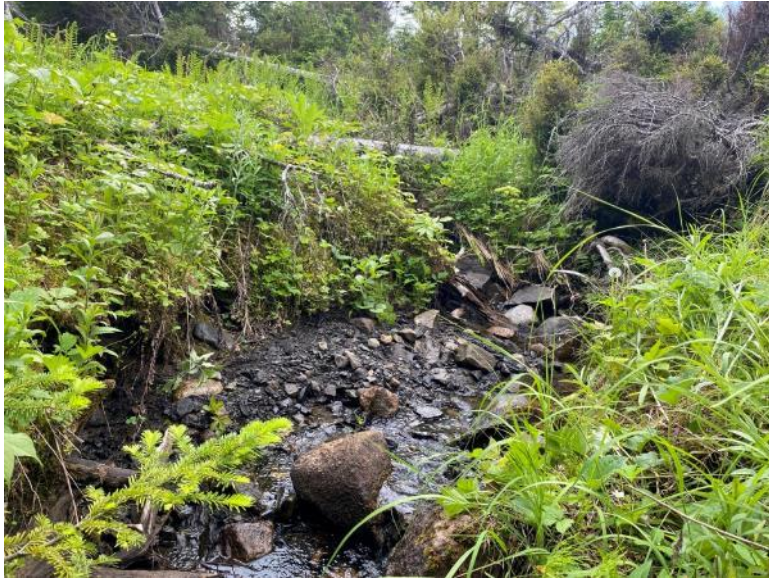
Photo 105 Watercourse Crossing WCA-074a Facing Upstream
