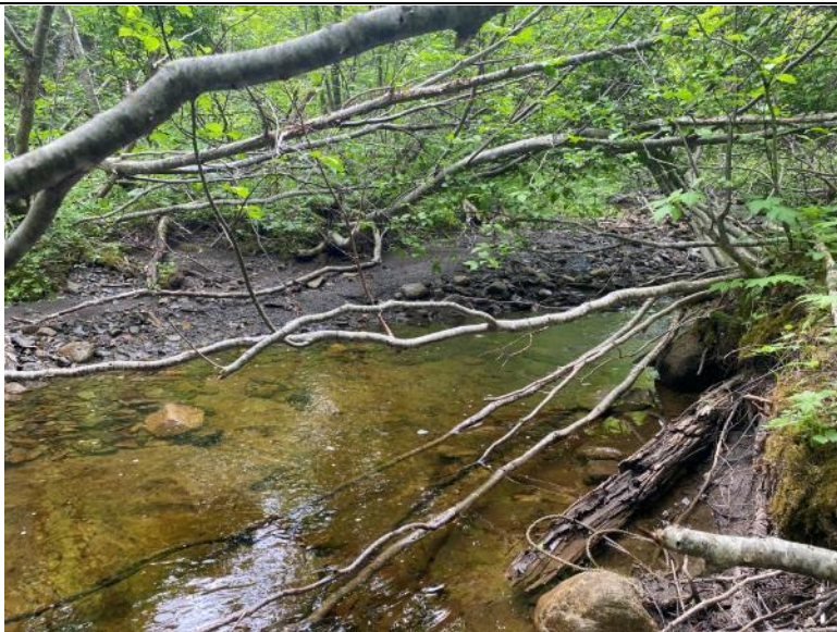
Photo 131 Watercourse Crossing WCA-110 Facing Upstream
