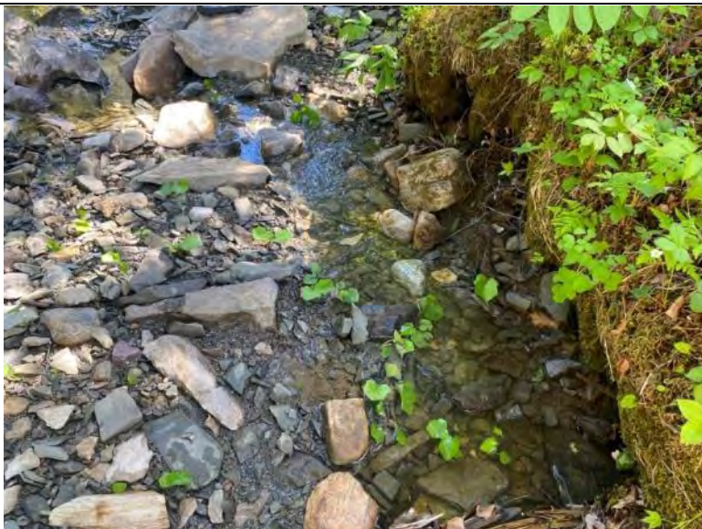
Photo 49 Watercourse Crossing WCL-719 Facing Upstream
