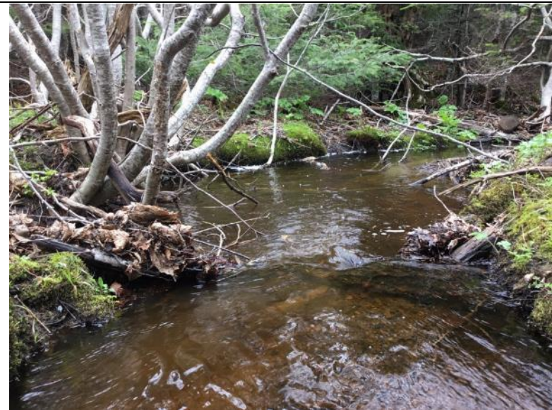
Photo 92 Watercourse Crossing WCA-071b Facing Downstream
