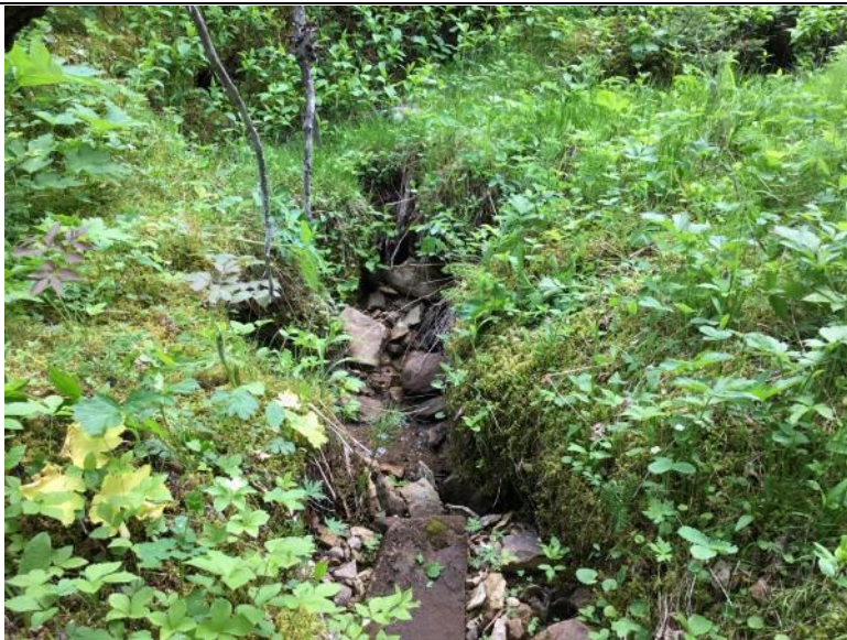
Photo 151 Watercourse Crossing WCA-123 Facing Upstream
