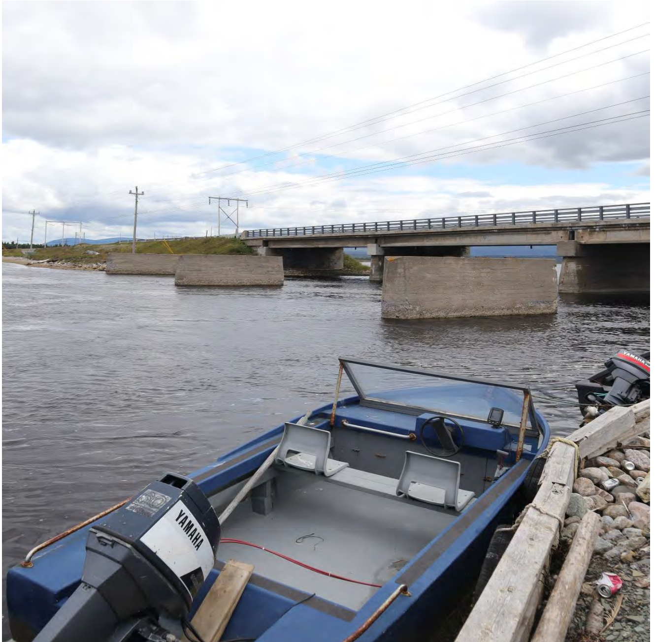
Figure 7. Existing Abutments of proposed Gateway Trail Head bridge
