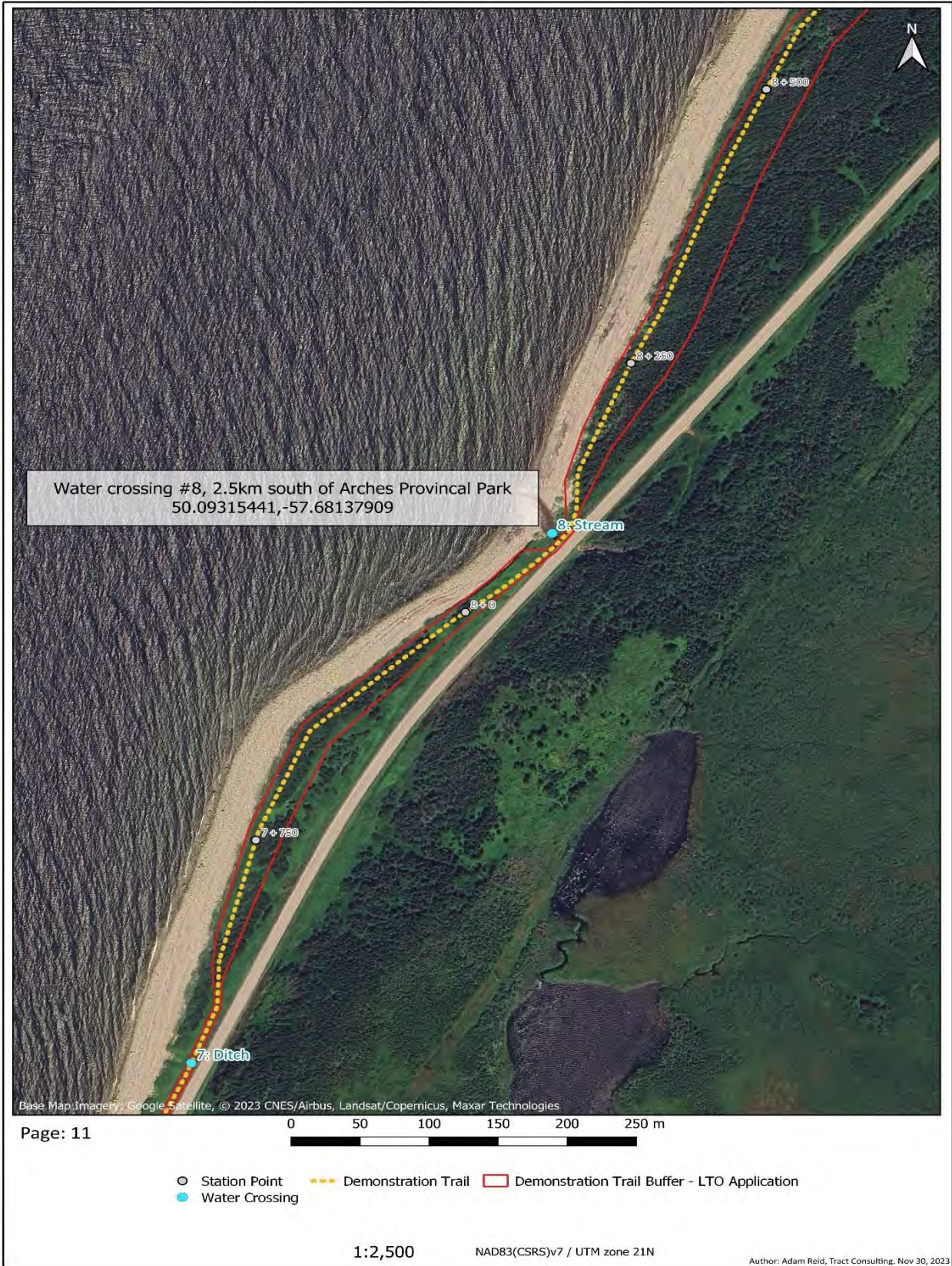
Figure 13. Location of water crossing #8, 2.5KM.south of Arches Provincial Park. Page 11 of the Demonstration Trail Map Book.
