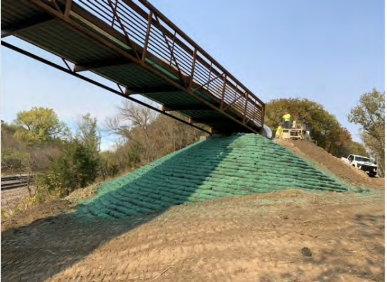
Figure 12. Example of Geotextile bag technology used as a bridge abutment.
