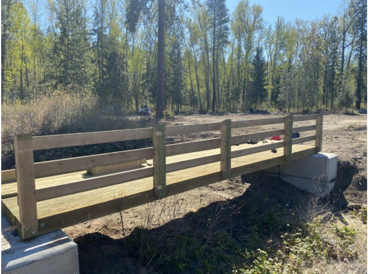
Figure 11: Example of a bridge design that will be similar to our crossing of Clam Cove river. Though Gabion cages will be used instead of cement for rock cribbing.
