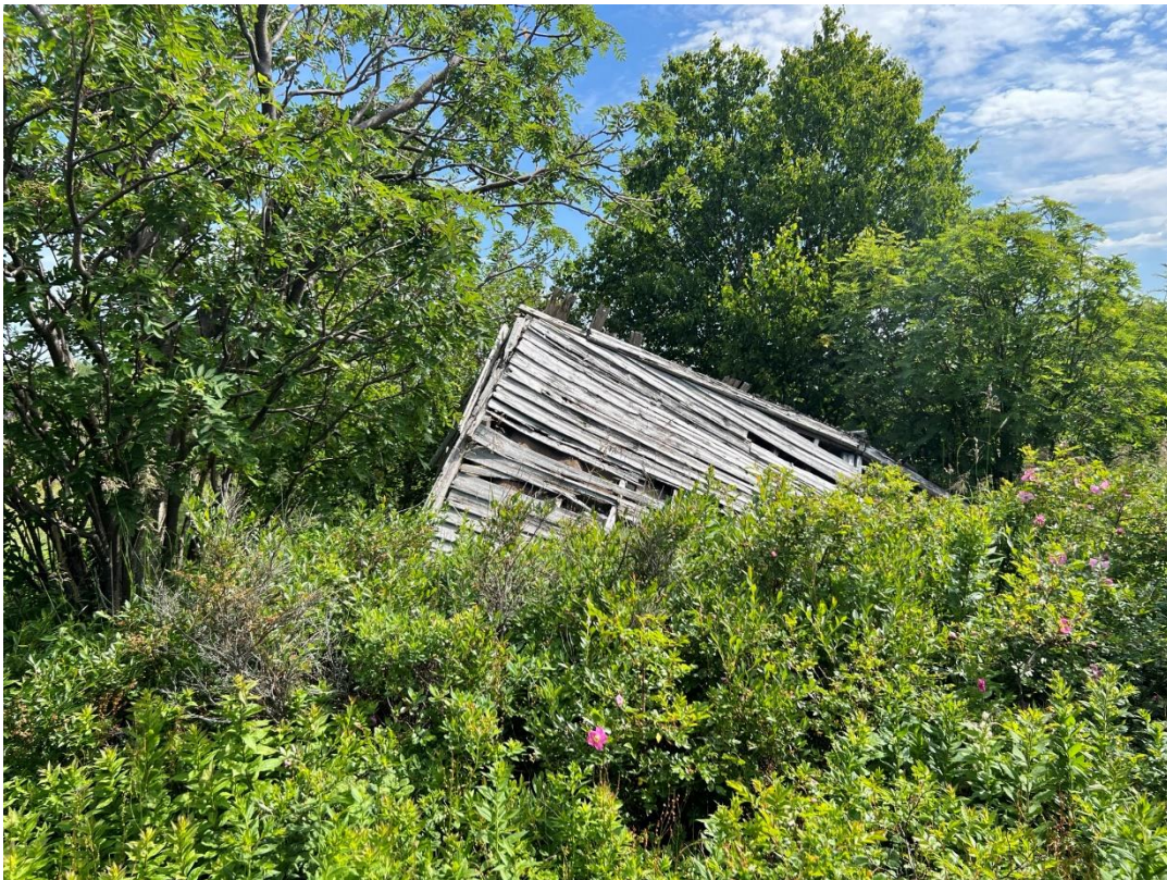
Photo 10.2: Dilapidated wooden structure found in Open Field Habitat
