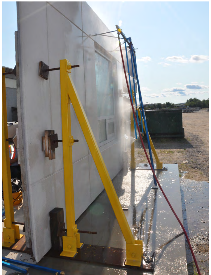
This image shows a window mockup being tested away from the construction site. Mockup testing can be a good way to verify functional performance and detailing before any related work is completed onsite.
