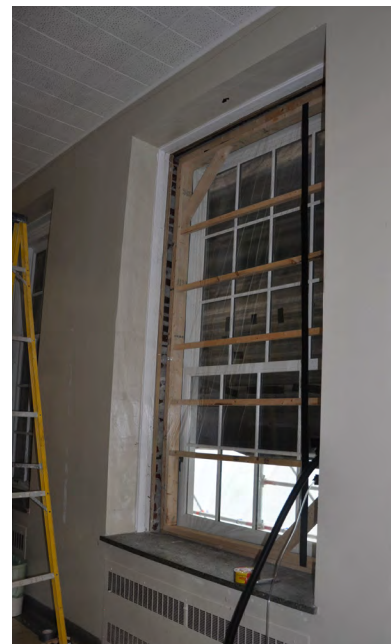
This image shows a window being tested for air leakage. The building owner was interested in learning whether the windows delivered and installed onsite met the expected performance ratings.
