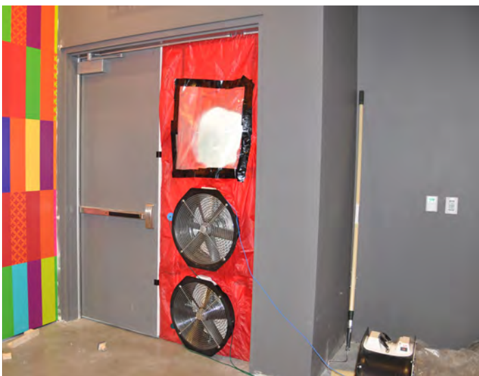
This image shows a functional performance test of a museum space's enclosed exhibit area. The client was interested in determining whether the contractor's air barrier installation met the specification in the construction documents.
