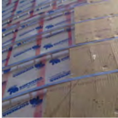
The "TcLip" from Engineered Assemblies. Source: Engineered Assemblies
