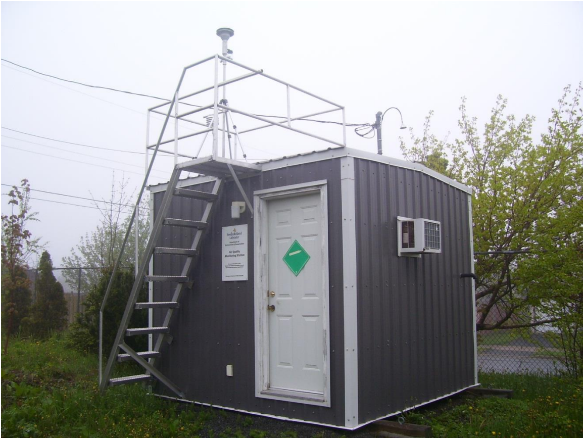
NAPS monitoring station in Mt. Pearl
