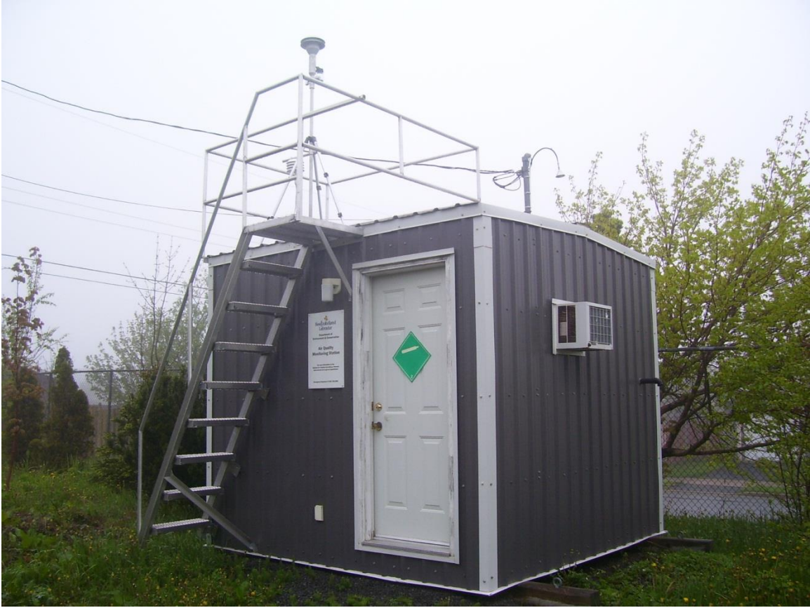
NAPS monitoring station in Mt. Pearl
