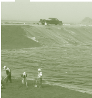
Installation of liner at Argentia demonstration hydrometallurgical plant.
