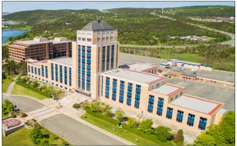
Confederation Building Complex, St. John's
