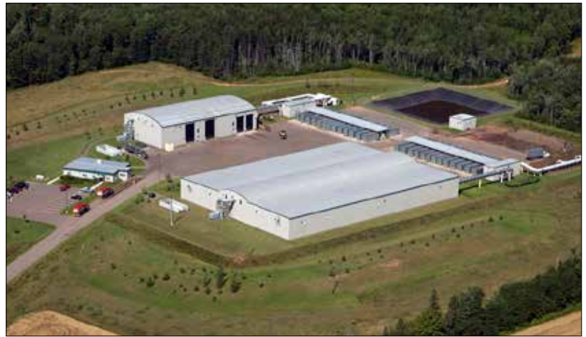
Central Composting Facility in PEI. Credit: ADI International (PEI)
