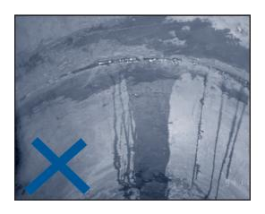
you can remove the lid with care. Inspect the inside casing using a strong flashlight. Look for holes or cracks, including evidence of animal infestations, or stains coming from the casing joints.
