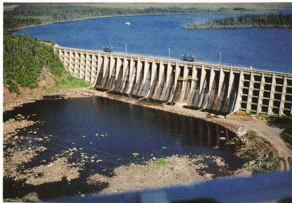
Figure 27.1 Large Hydro Dam on Deer Lake
