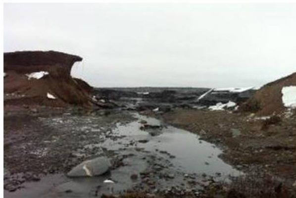
Gullbridge mine breach in December 2012.
