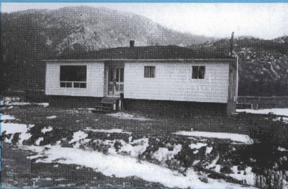
The same house after being elevated.
