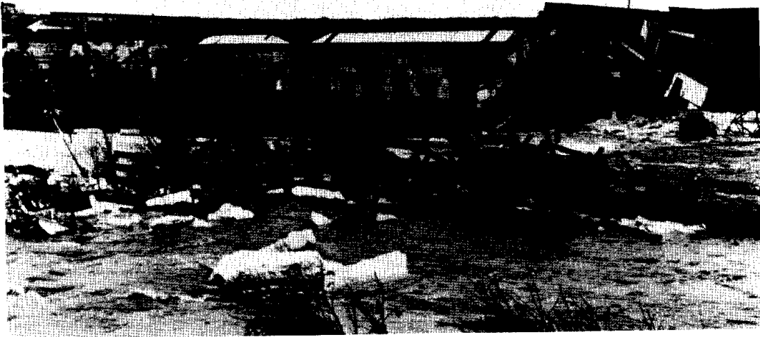
Photograph 7.4 - Old Groundwood Mill at Bishop's Falls beginning to collapse, early afternoon, January 14, 1983
