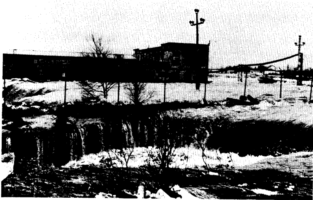
Photograph 7.2 - Old Greenwood Mill at Bishop's Falls prior to collapse - midday on January 14, 1983
