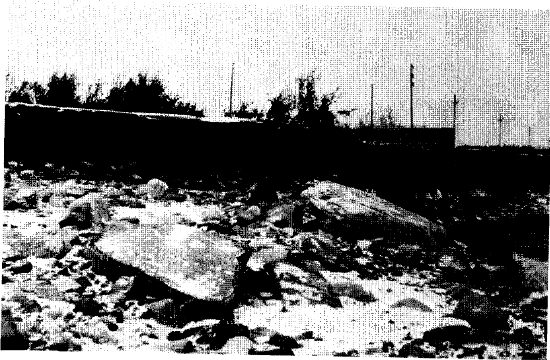
Photograph 7.10 - Downstream End of Bank Erosion, Bishop's Falls - January 14, 1983
