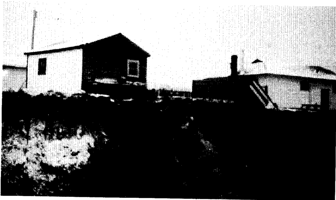
Photograph 7.11 - Eroded Bank along New River Channel
