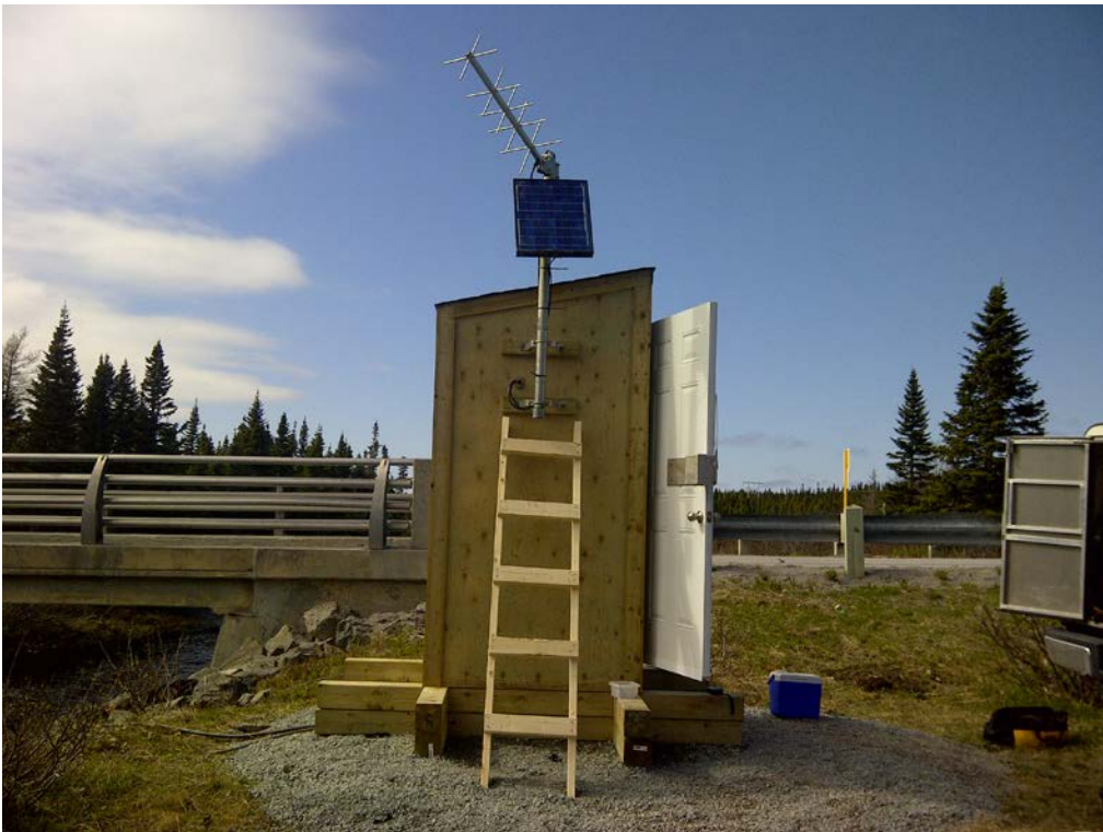
Bartlett's River after the reconstruction
