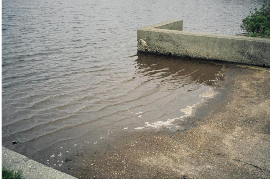
Plate 9 – Waterford River at Bremigan’s Pond – Outlet Structure
