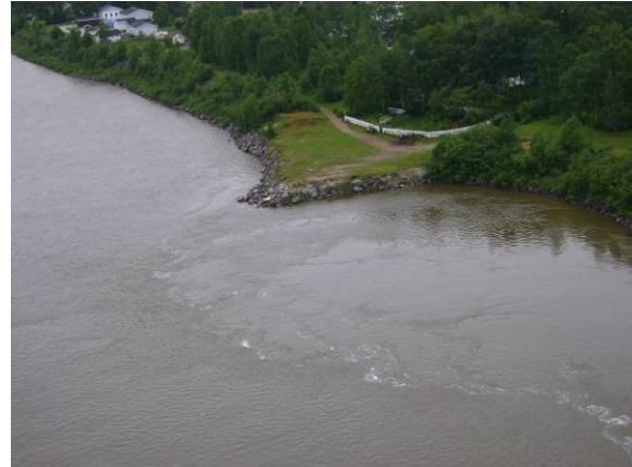
Photo 3 - Lower Outfall (Corte Real Rd)
