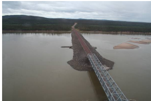
Photo 1 – Trans Labrador Highway Bridge and Causeway over Churchill River
