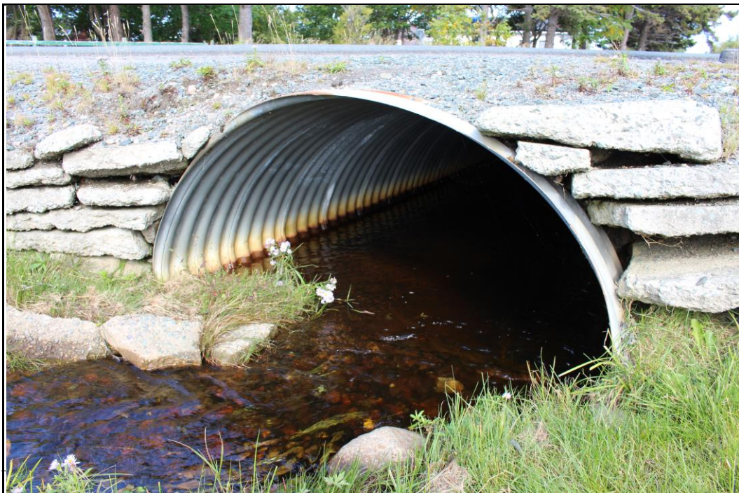
Figure 5.3 Corrugated Steel Arch Culvert
