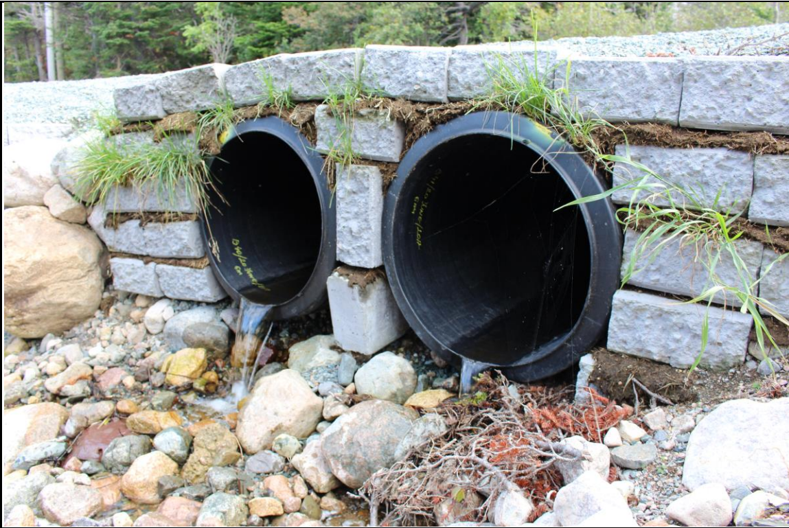
Figure 5.8 Two Culverts with a Shared Outlet Location
