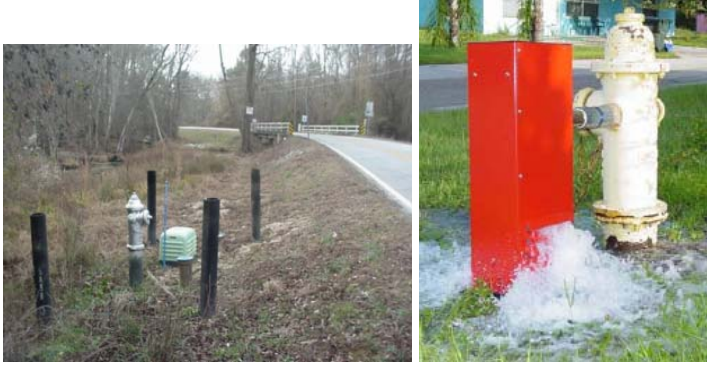
Figure 36: Hydro-Guard automatic flushing devices
