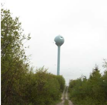
Figure 138: Hawke's Bay water storage tank
