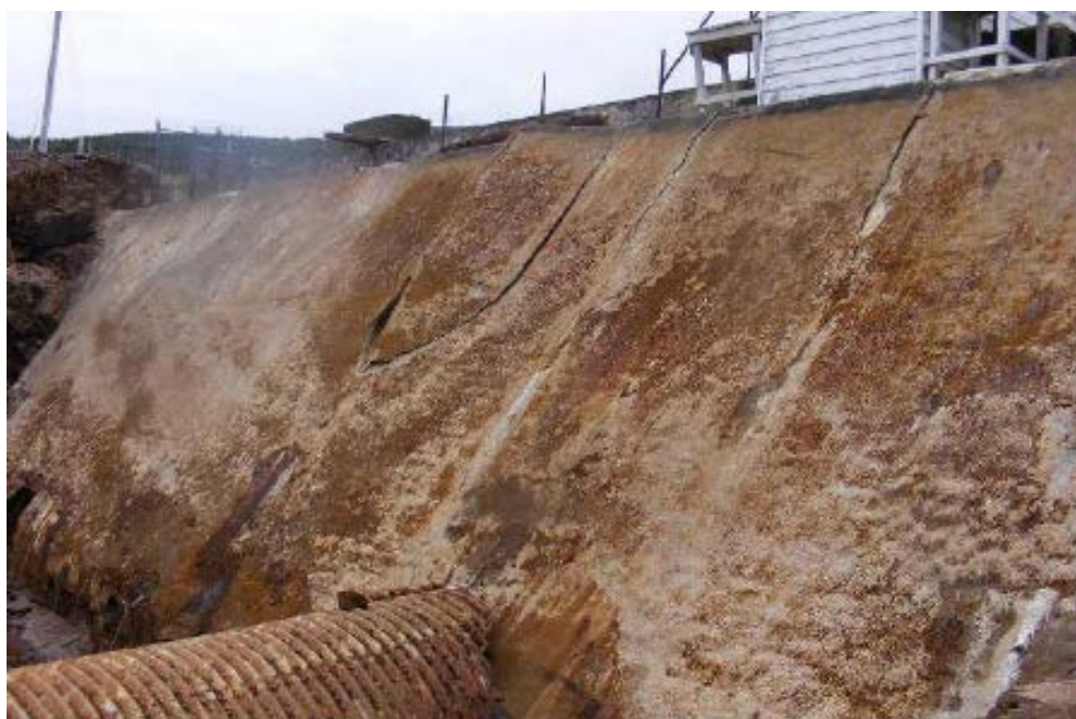
Figure 26: Lawn Forebay Dam - showing cracked and displaced concrete.
