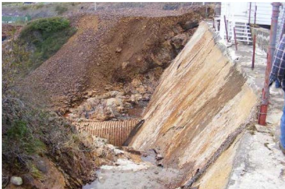
Figure 25: Lawn Forebay Dam – showing eroded abutments.
