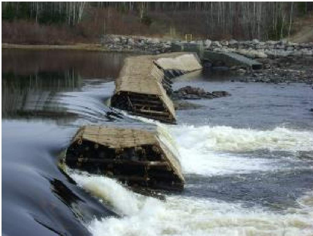
Figure 1: Goodyear's Dam – showing the two failed sections.
