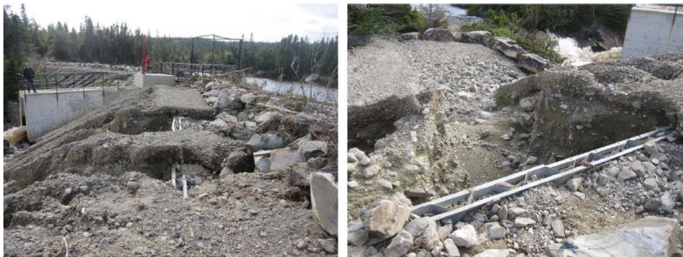
Figure 28: Port Union Hydroelectric Development - showing erosion along the dam and the dam's steel core.
