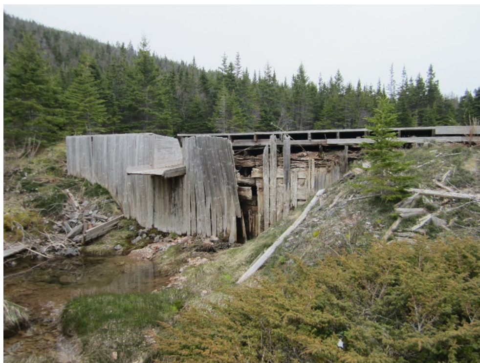
Figure 8: Sheaves Cove Dam – showing deterioration of the downstream side of the main dam.
