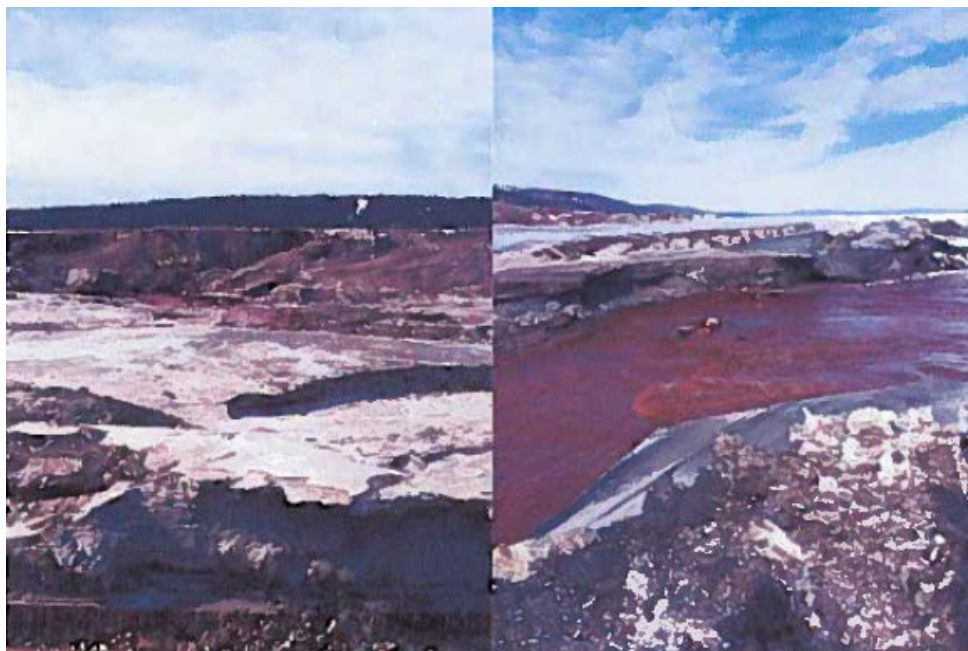
Figure 21: Central Control Dike – showing extent of the failed tailings.
