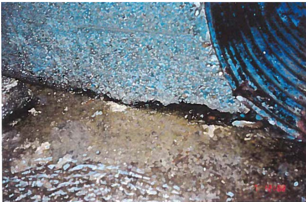
Figure 3: Dam 1 (Merrymeeting Pond) - cracking in spillway
