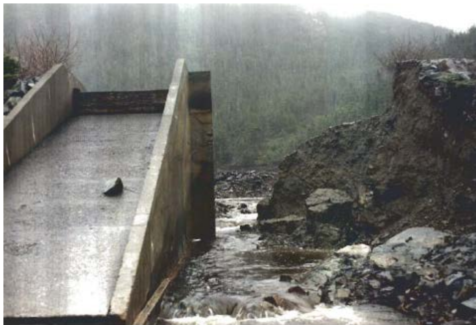
Figure 31: Granfer's Pond Dam – showing showing the dam washout and the stoplogs in the spillway.
