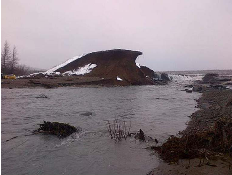
Figure 15: Gullbridge Tailings Dam – showing the breached section.
