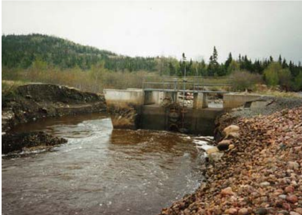
Figure 30: Bully's Pond Dam - showing the dam failure in 1995.
