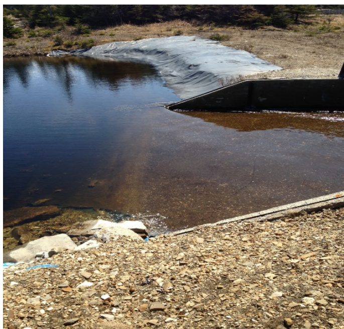
Figure 13: Well Cove Brook Dam showing spillway on the upstream side.
