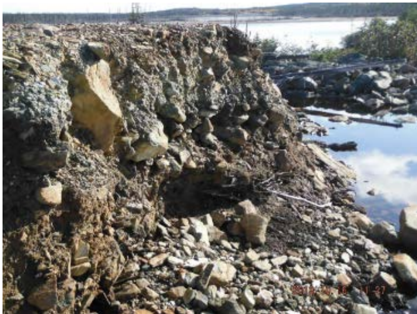
Figure 19: West Dam – showing the material within the dam.
