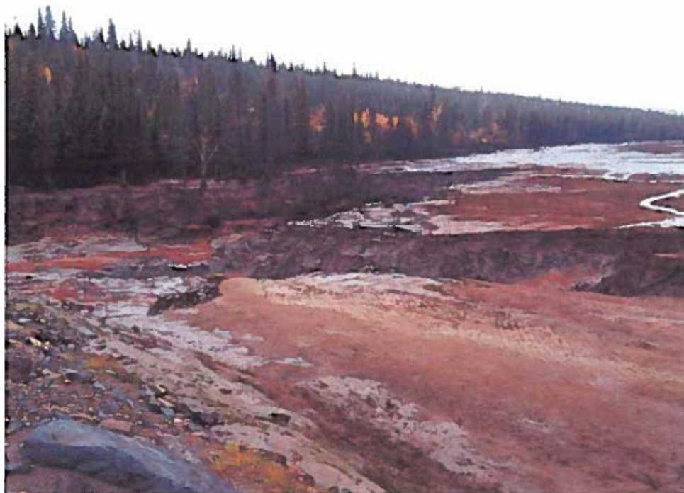
Figure 23: Jody's Dike – showing the extent of the 2012 breach.
