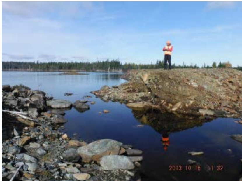
Figure 18: West Dam – showing the breached section.
