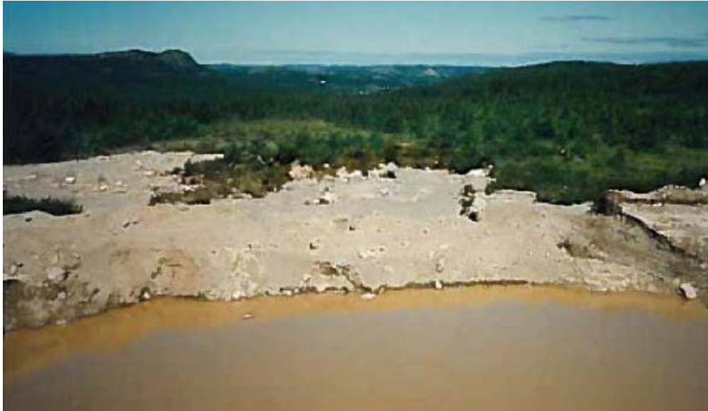
Figure 34: Concrete Products Berm – showing section of the berm that breached.
