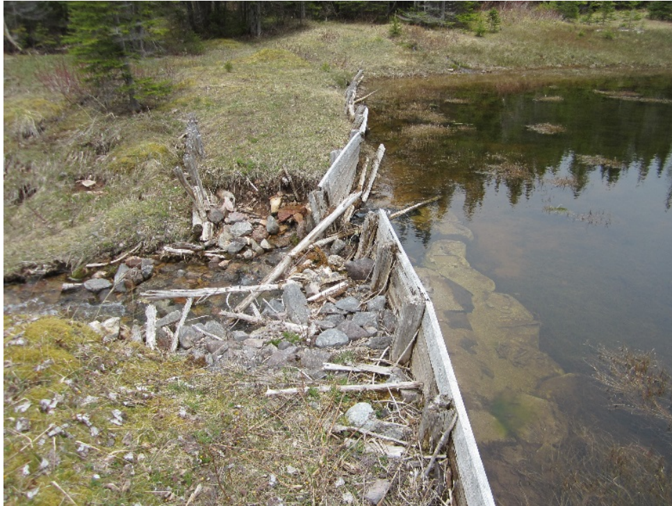
Figure 9: Sheaves Cove Dam – showing the small reserve dam and failed area.
