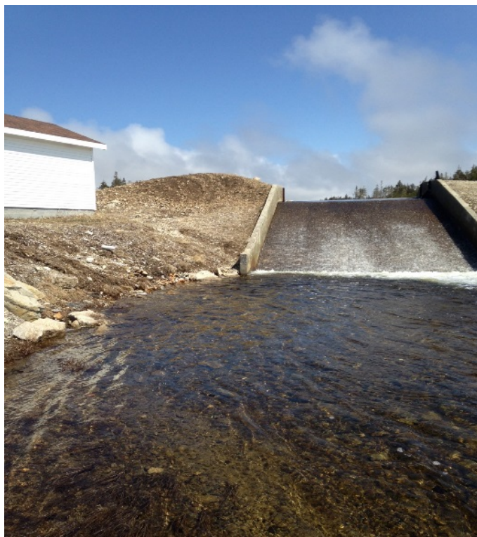
Figure 12: Well Cove Brook Dam – showing spillway (photo 2).
