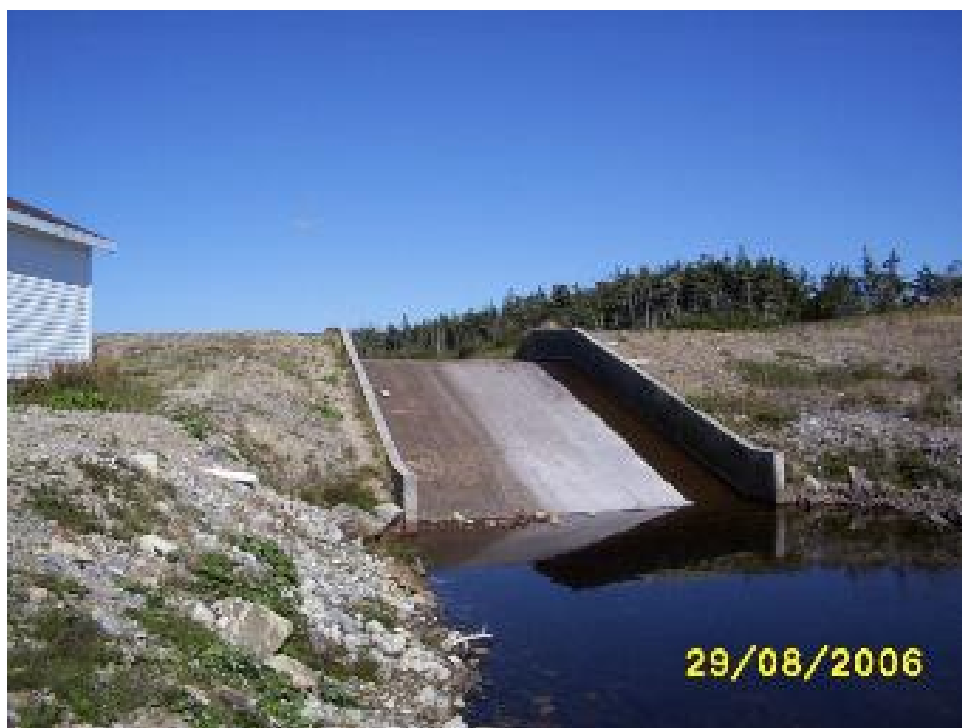
Figure 11: Well Cove Brook Dam – showing spillway (photo 1).
