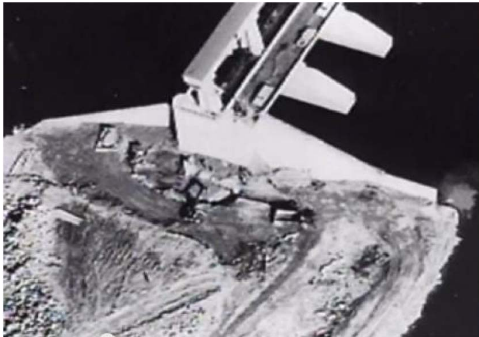
Figure 14: Dike GJ-11A – showing aftermath of the washout.
