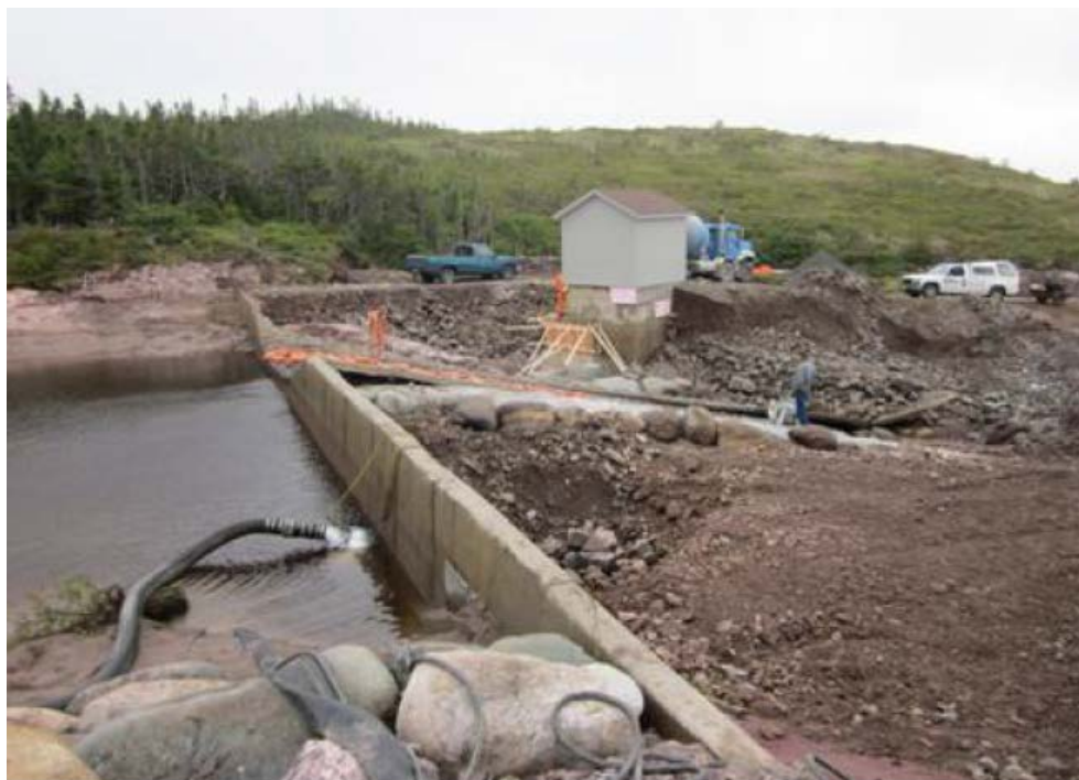
Figure 29: Sunnyside Water Supply Dam - showing damage to the dam.
