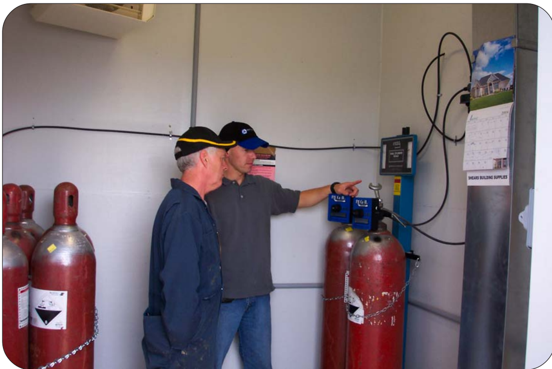
Operator Trainer Gerry Lahey (right) providing training to Pasadena water system operator Chris Upshall (left) on their gas chlorination disinfection system.
