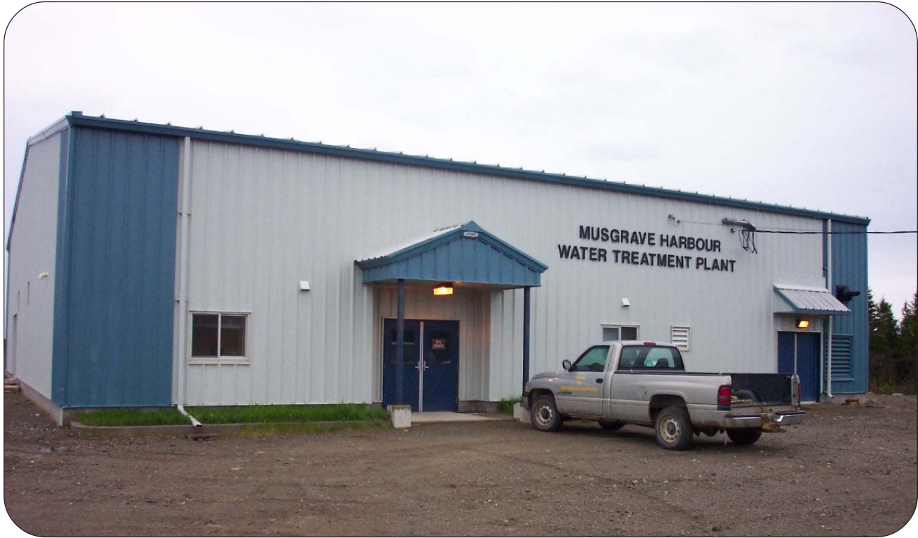
The Musgrave Harbour water treatment plant. This is a conventional packaged water treatment plant that was installed in 1998.
