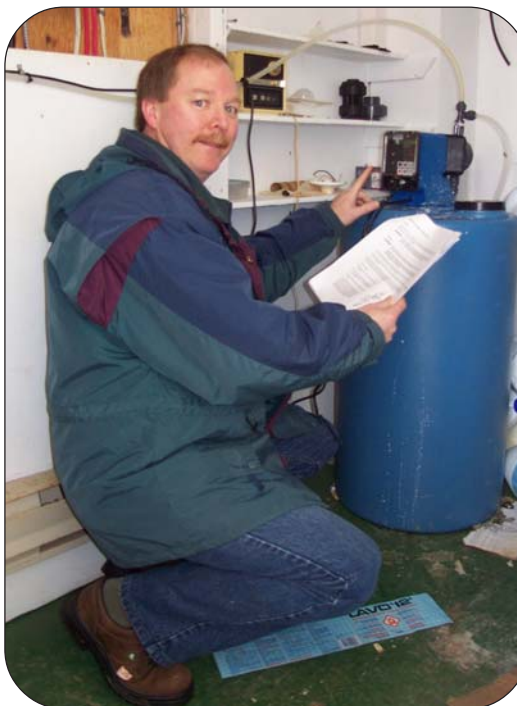
Water and Wastewater Specialist Ron Goulding inspecting a hypochlorination unit in the community of Lawn.
