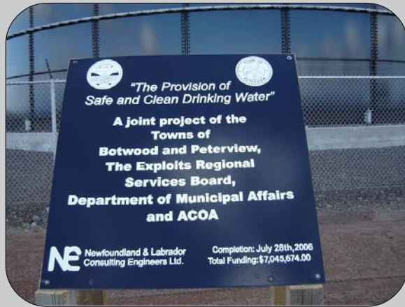
Plaque announcing the new regional supply with the storage reservoir in the background.
