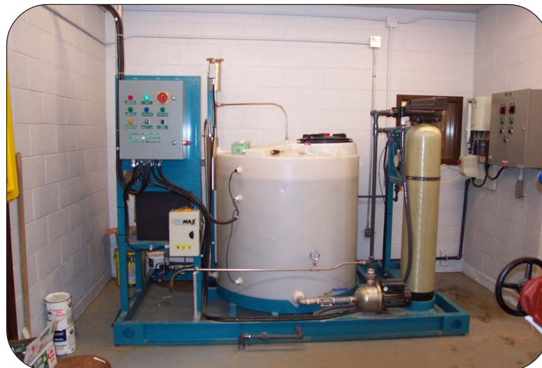
Small-scale treatment unit in the central Newfoundland town of Buchans.
