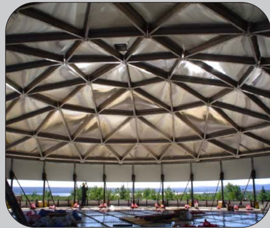
The interior of the storage reservoir.
