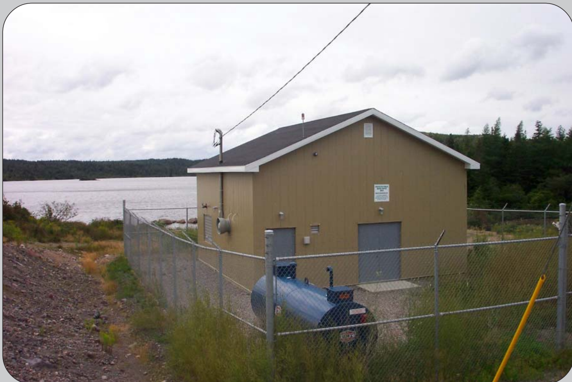
Avondale chlorination building with Lee's Pond supply pond in the background.
