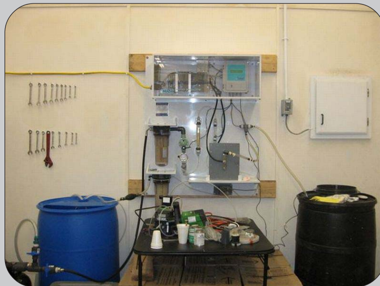
Above: The MIOX Disinfection System in Heart's Delight–Islington.
