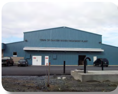
Water Treatment Plant - Gander
