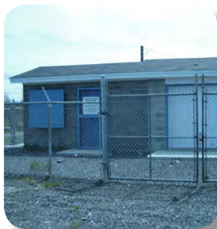
Chlorination Building - Spaniard's Bay
