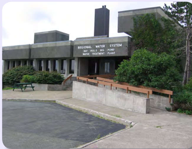
Bay Bulls-Big Pond Water Treatment Plant (Photo Credit: Lynnann Stapleton)
