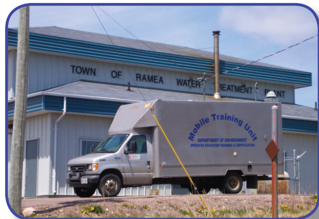
The Department's MTU outside the Ramea Water Treatment Plant
