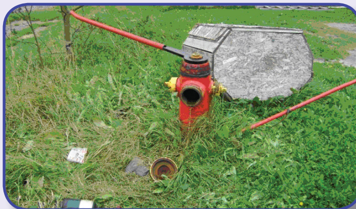
Hydrant under repair
