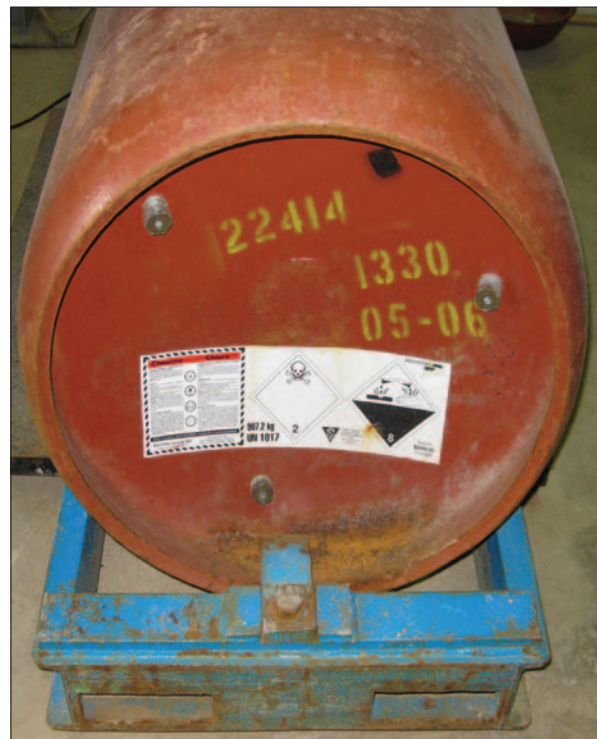
Chlorine gas tonner, Channel - Port aux Basques Water Treatment Plant, Newfoundland
