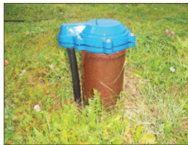
Example of open well and well with vermin proof cap
