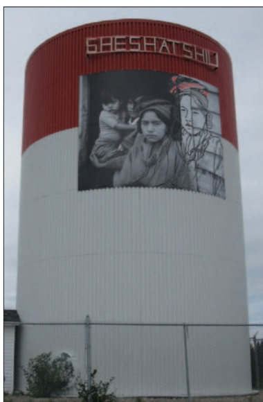
Water storage tank, Sheshatshiu, Labrador
