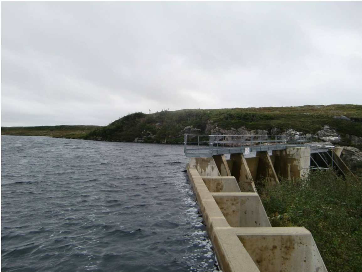
Figure 5.6 Dam system on the Community C water supply
