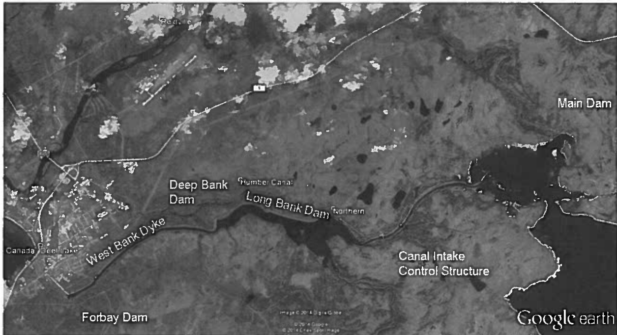
Figure 5: Deer Lake Power System
