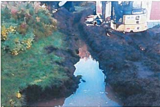
Figure 4: Western Star photo- Richard Dewey took this picture of the trench he dug in his yard to show the town how properties around the Deer Lake canal are being flooded
