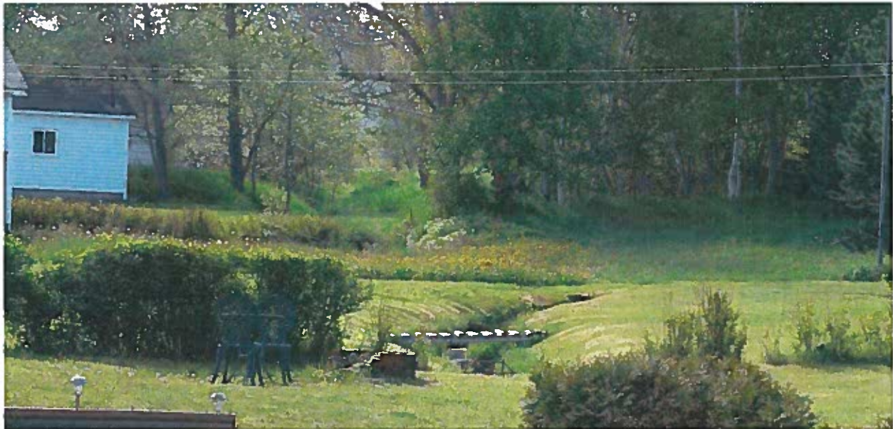
Figure 8: South stream running through backyards of homes on Main Dam Rd. before entering town's stormwater system (see extended edge of metal grate across drainage culvert)
