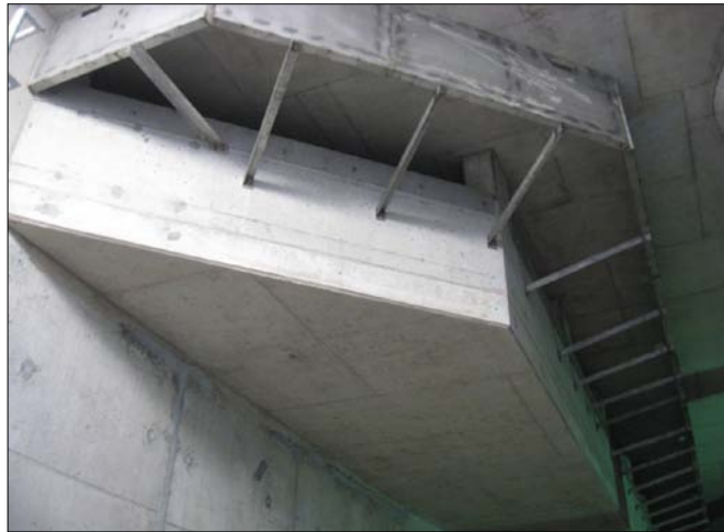
Figure 6-44 - Underflow Baffle on CSO Tank Overflow (Hamilton, Ontario)
