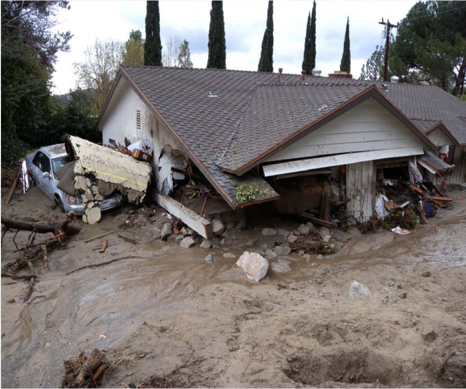
Post Wildfire Debris Flows, 2009 Station Fire, CA (USGS)
