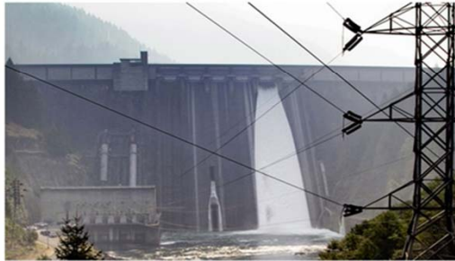
Detroit Dam, southeast of Salem, Ore., on the North Santiam River, provides a variety of functions including flood risk management and power production. However, it also blocks fish passage and the U.S. Army Corps of Engineers is in the process of building temperature control and fish passage at this site.
