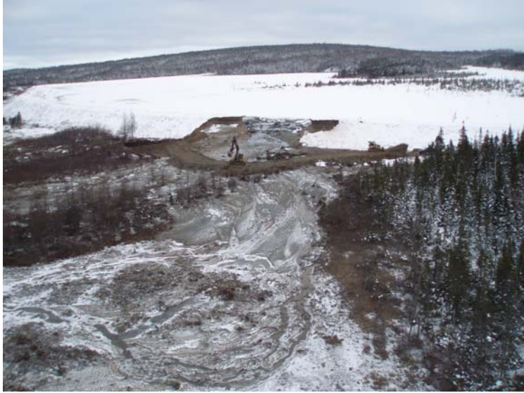
Picture #7: Section of bog immediately downstream of breach
