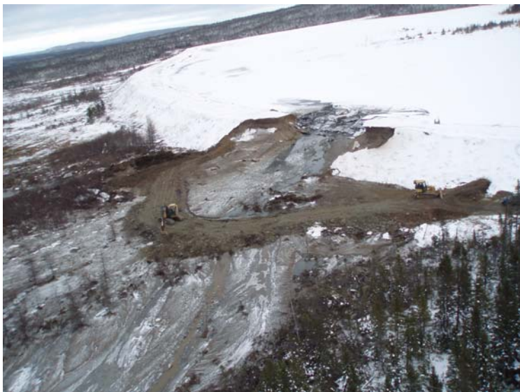
Picture #8: Construction of berm for temporary containment and settling pond
