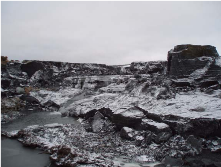
Picture #2: Consolidated tailings at breach outlet
