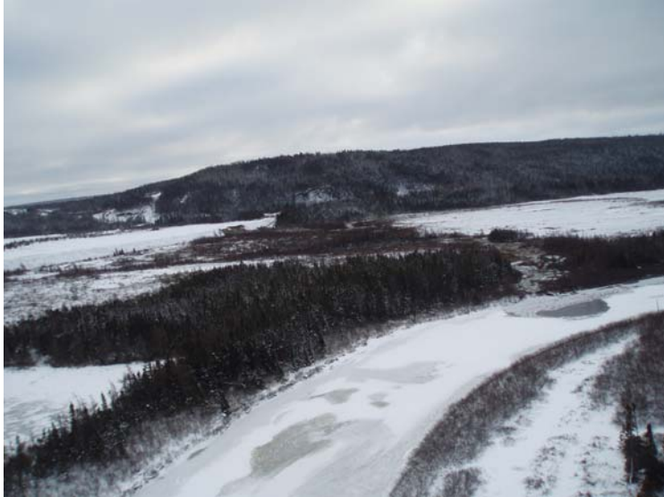
Picture #3: Breach water enters South Brook, with dam in background
