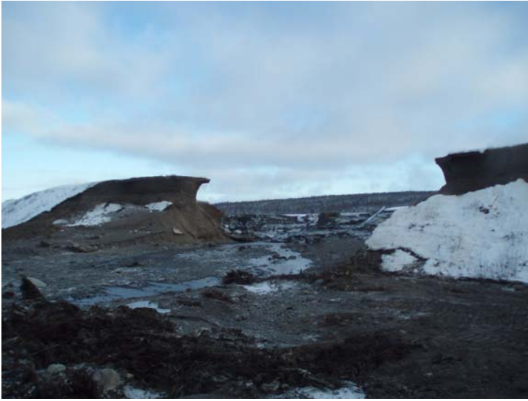
Picture #1: Gullbridge Breach
