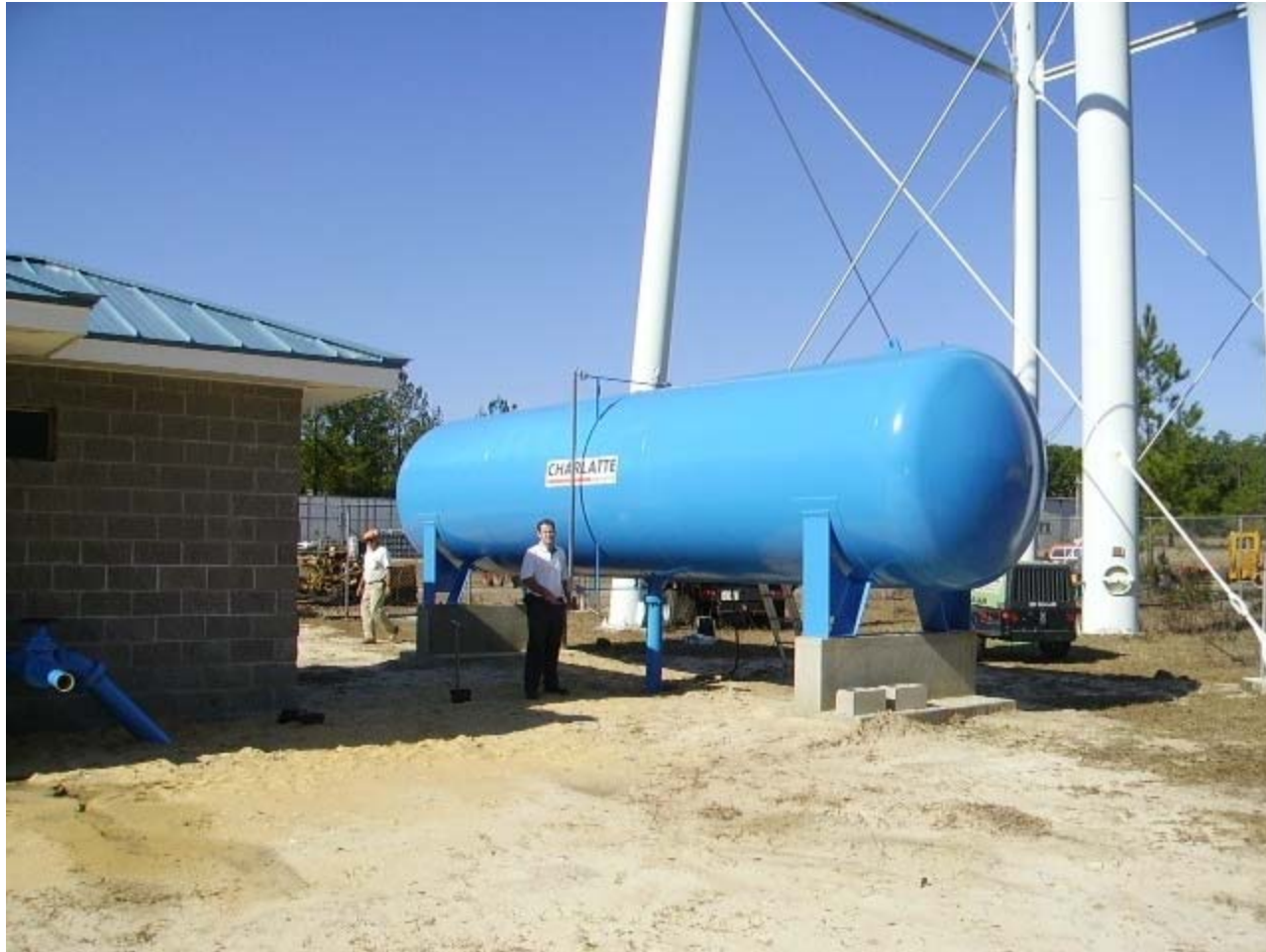
Hydrofort 7925 gallon bladder type hydro vessel Florida
