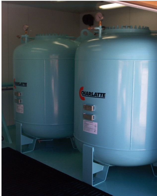
TAZEWELL COUNTY PSA TAZEWELL COUNTY, VIRGINIA. 2x400 GALLON POTABLE WATER BLADDER VESSELS.
