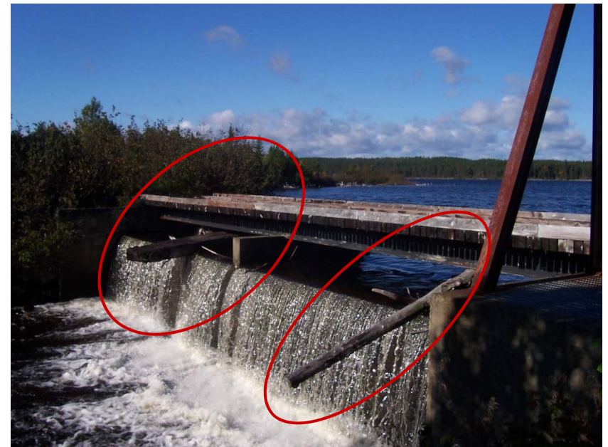
Debris blocking spillway
