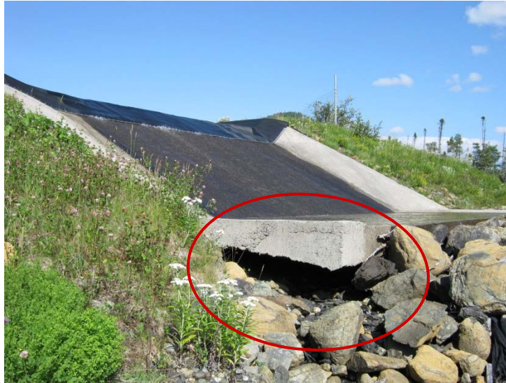
Scour and erosion at base of spillway
