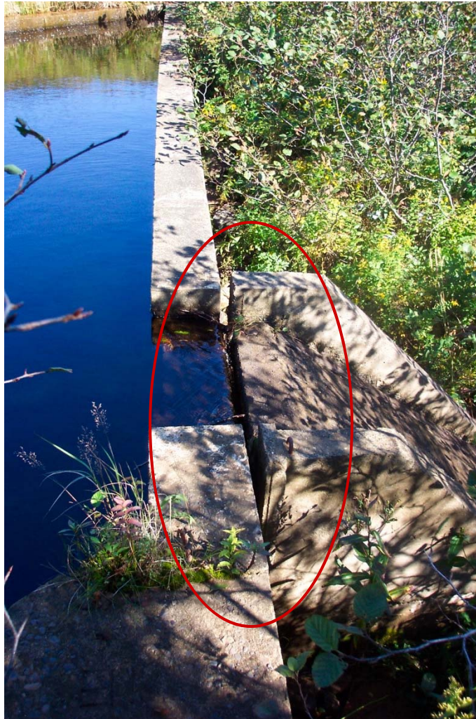
Concrete structures out of alignment
