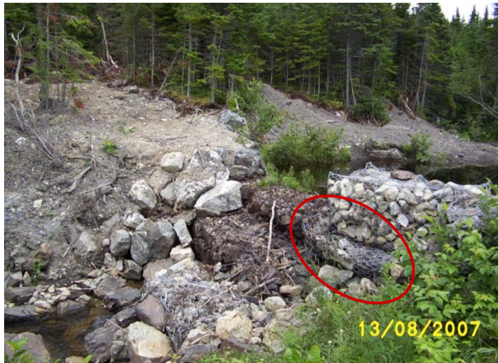
Deteriorating timber cribbing and gabions
