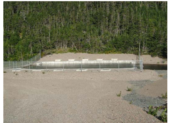
Finished Infiltration Gallery
