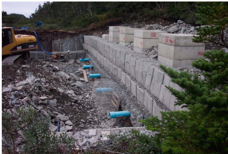
Construction of Buried Infiltration Gallery
