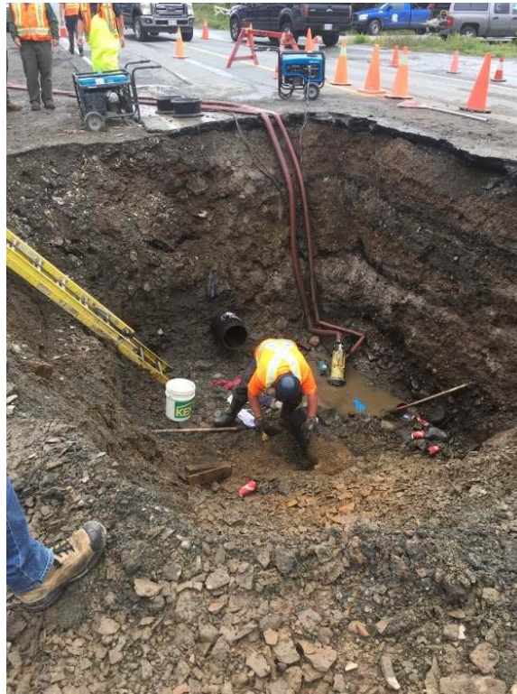
Water main repairs
