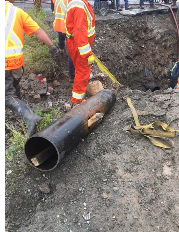
Section of 12" DI water main removed
