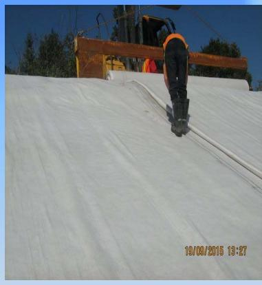
Placing bentonite sealant between horizontal and vertical joins in GCL liner. Once contacted with water the bentonite will expand creating a waterproof seal between the layers.
