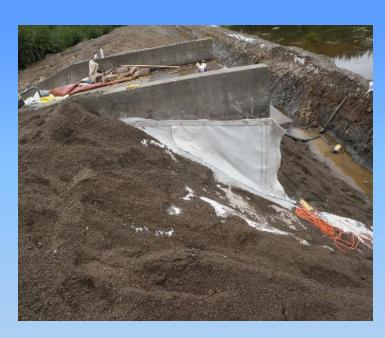
Tying in the GCL liner to seal around the 400 mm drain pipe and the concrete face of the spillway structure. Proper installation is crucial to getting a water tight seal.
