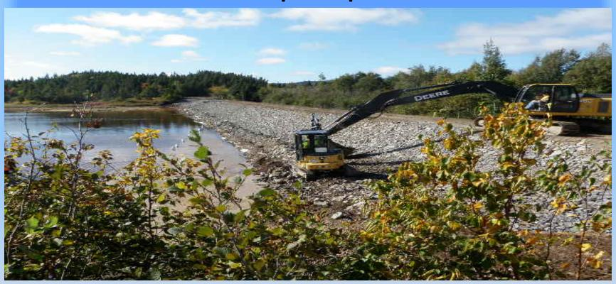
Two excavators working in tandem to complete rip rap placement at the toe of the upstream slope.
