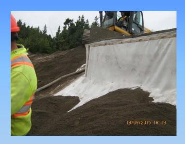
Maintaining waterproof seal around the spillway structure
