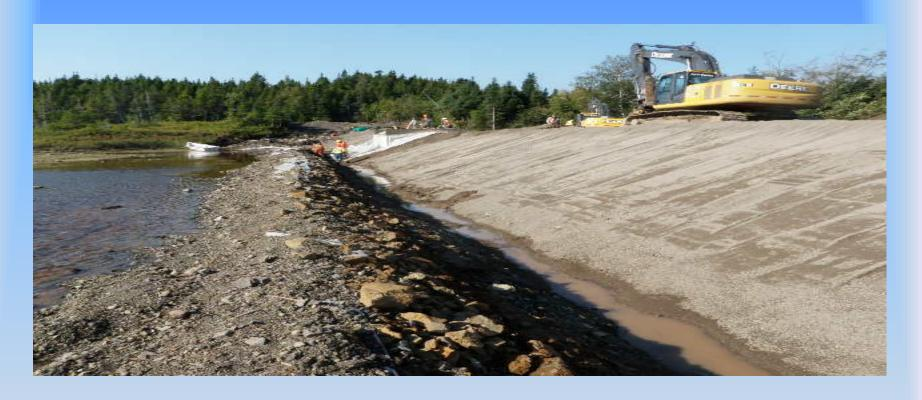
Here you can see a large section of the upstream dam face prepared for the installation of the liner. The slopes have been dressed to 3:1. A uniform sand and gravel bed has been compacted in place.
