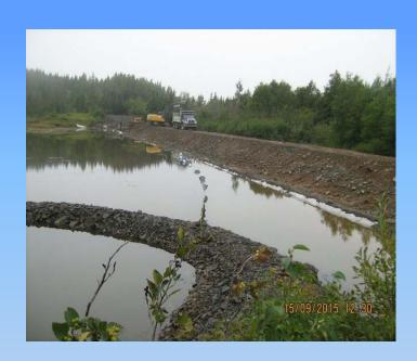
Excavating and hauling away overburden while shaping dam slopes:
