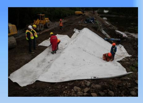
Working on section between far shore and spillway. The first picture shows the slopes prepared for Geosynthetic Clay Liner (GCL). The second picture shows the liner being installed up to the top anchor trench.
