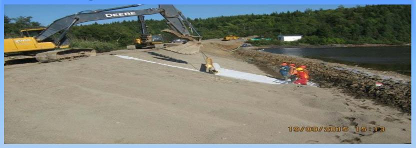
Installation and covering of the GCL liner is shown here.
