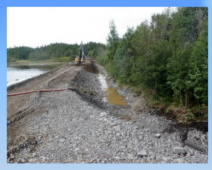
This is how the dam looked after completion of the grubbing on both slopes.
