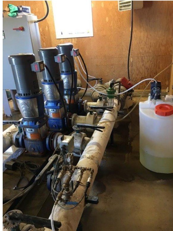
Liquid Chlorine Injection System
