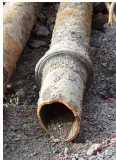
Cast iron pipe from 1960s
