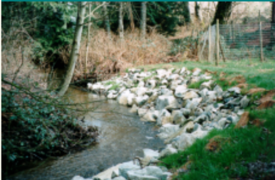
Stream bank protection
