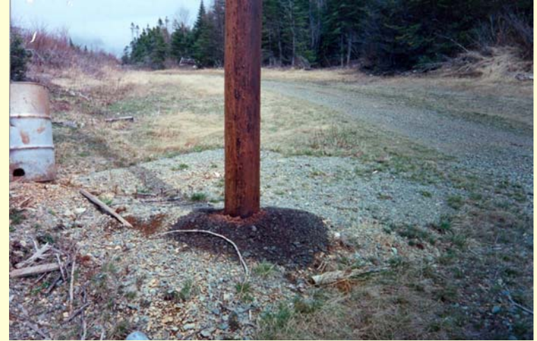
Creosote draining out of pole in Beachside
