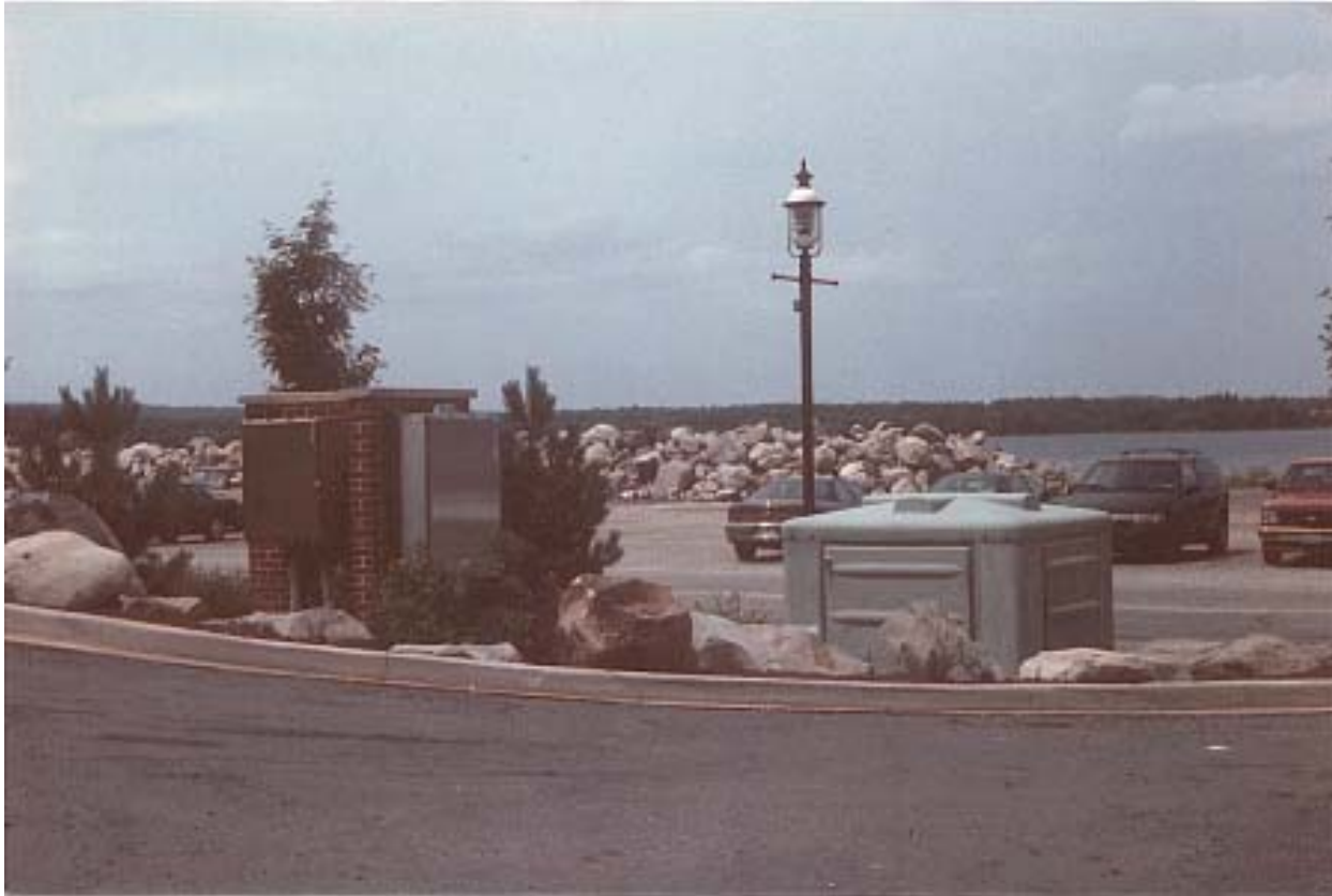
Town Of Liverpool Pumping Station
